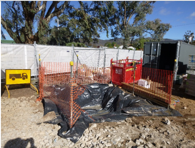
Photo 3 – Concrete washdown area rectified
