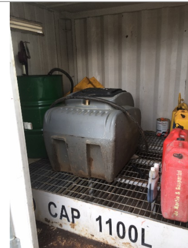
Photo 4 – Oil tank put back in the hazardous substances' container
