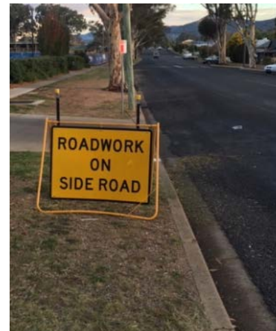
Photo 8 – TCP and Traffic Control sign in place
