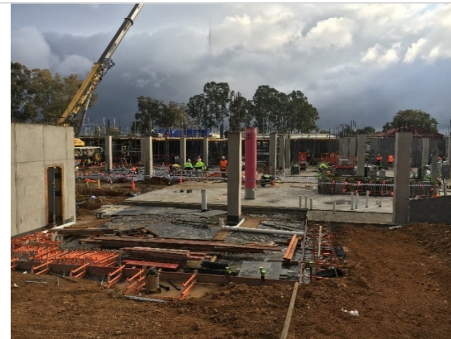
Photo 16 – Crane operations and concrete works
