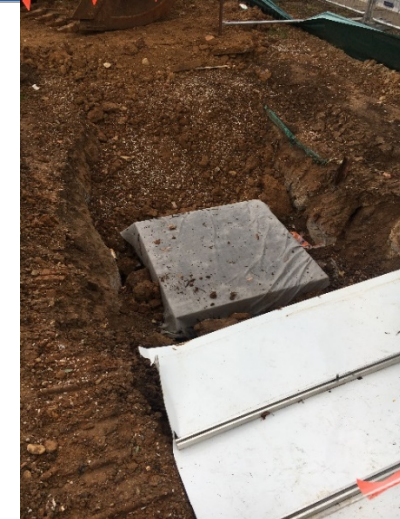
Photo 6 – Erosion and Sedimentation Controls in place
