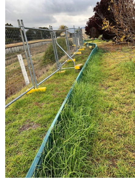
Photo 14 – Silt fence around stockpile are well installed and maintained
