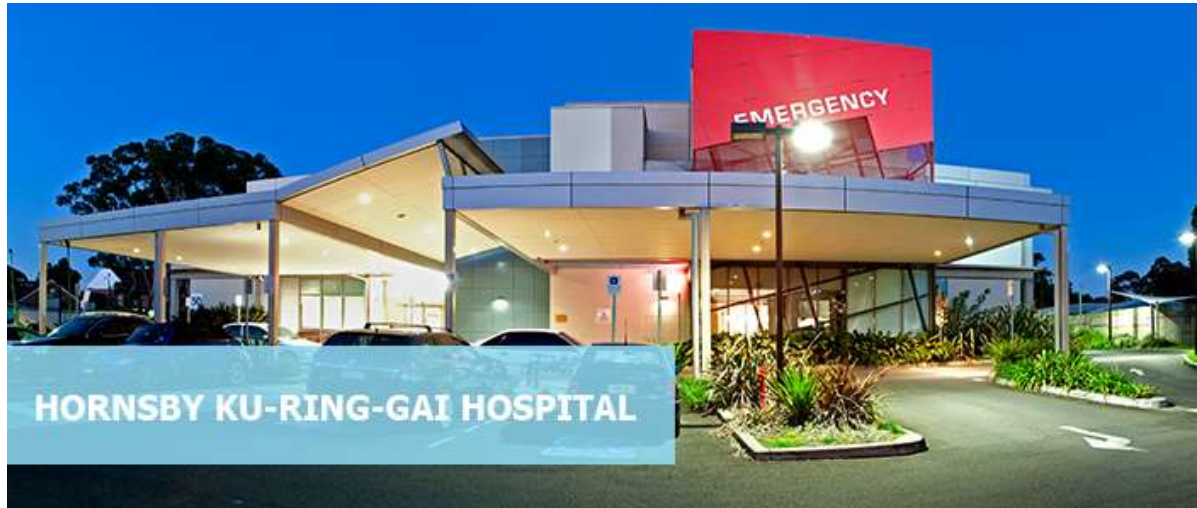
Existing Hospital Main Entry / Emergency Department (Palmerston Road)
