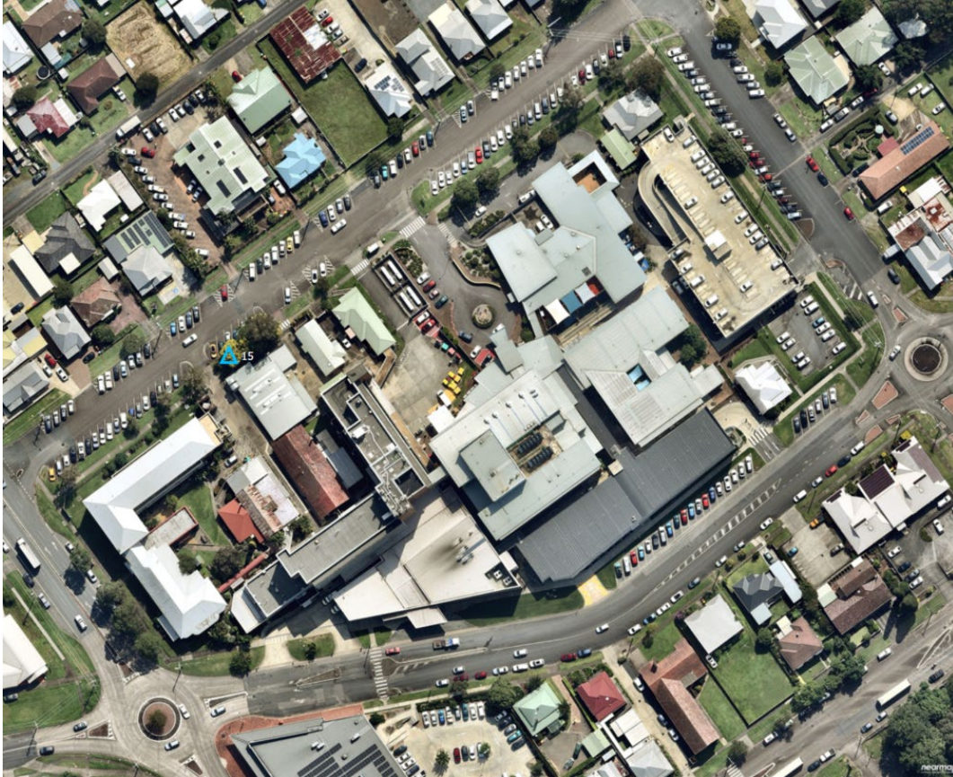
Figure 9. Site map showing tree requiring specific protection measures. (ArborSafe, March 2022).
