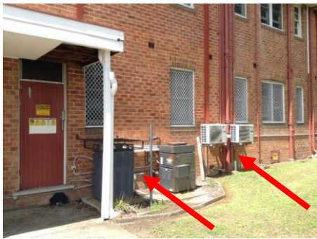
Photo No. 014: Subfloor of Eastern Wing
