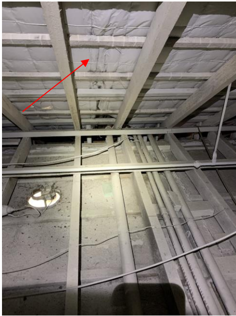
SMF – Foiled back insulation Level 01 “west wing”
