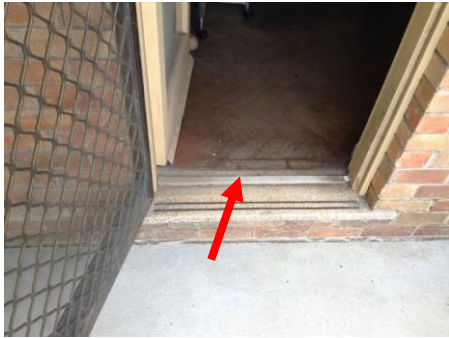
Photo No. 001: South-western entrance
