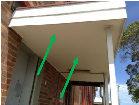
Photo No. 018: Entry Portico (off Room MN0900037)
