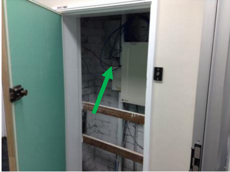
Photo No. 024: Ground Floor Room MN090027
