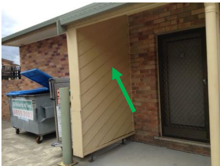
Photo No. 008: South-Western Entrance
