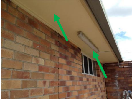
Photo No. 007: Front Extension
