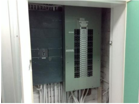
Photo No. 013: Ground Floor Room MN090028
