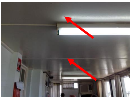
Photo No. 009: Ground Floor MN0900063
