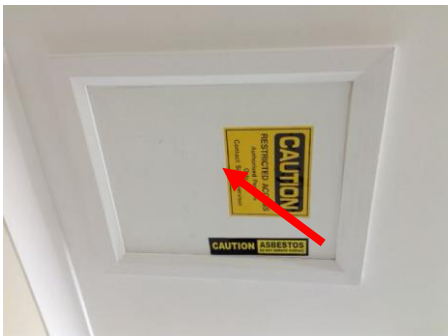
Photo No. 006: Ground Floor, men's bathroom MN0900044
