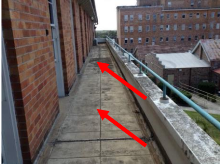
Photo No. 004: 2nd floor eastern balcony
