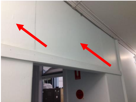
Photo No. 005: Ground Floor, bulkhead outside MN0900059
