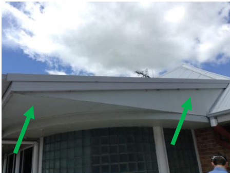
Photo No. 019: 1st Floor Eaves
