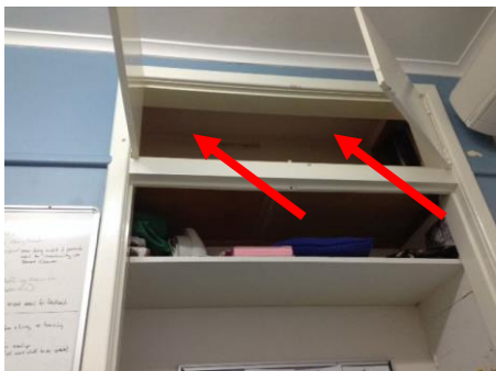
Photo No. 015: 1st Floor, upper cupboard to Room MN0901039
