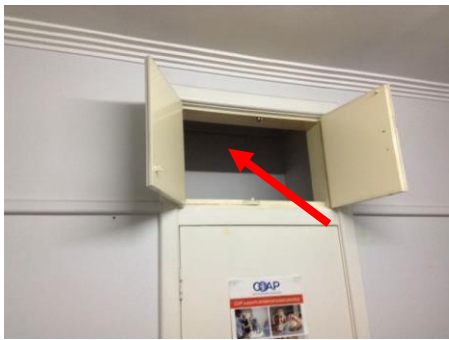
Photo No. 017: 1st Floor, upper cupboard to MN0901042
