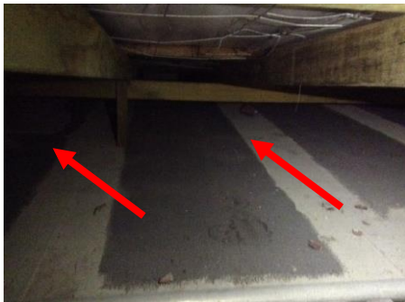
Photo No. 002: 1st Floor Ceiling Void
