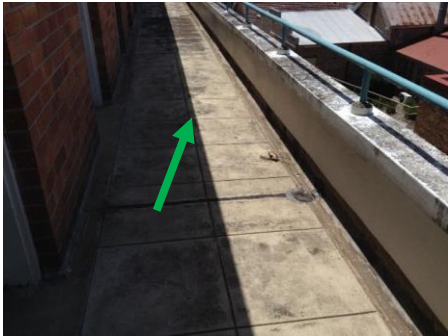
Photo No. 021: 2nd floor Eastern Balcony
