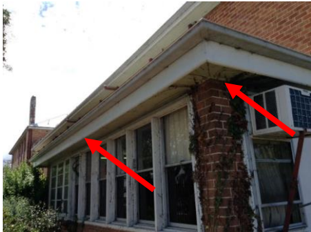
Photo No. 008: Eave soffit outside room MN0900056
