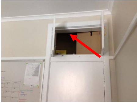
Photo No. 016: 1st Floor, upper cupboard to Room MN0901040 and MN0901041
