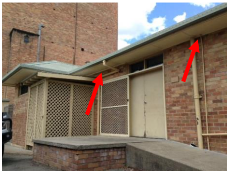
Photo No. 002: Original building
