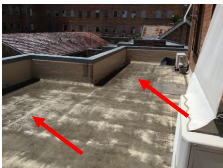
Photo No. 003: 1st floor north east balcony
