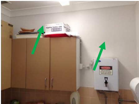
Photo No. 022: Ground Floor Room MN090010
