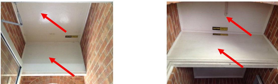
Photo No. 012: Ground Floor, North Eastern Entrance Alcove
