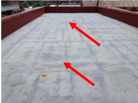
Photo No. 001: 1st Floor Balcony (above Staff Centre)
