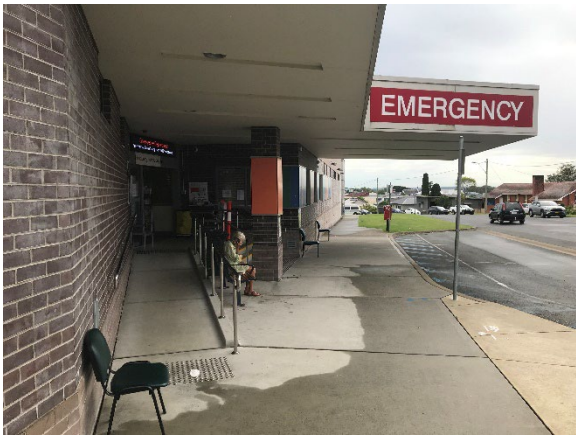
Plate 6.5 View east showing hospital buildings and hard surfaces in SU2
