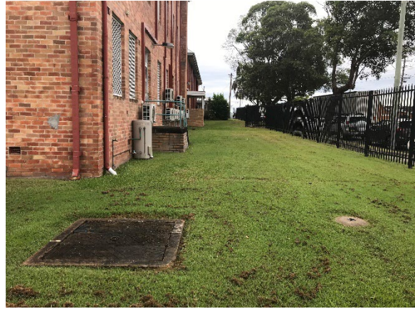
Plate 6.4 View south-east showing evidence of subsurface services along Commerce Street
