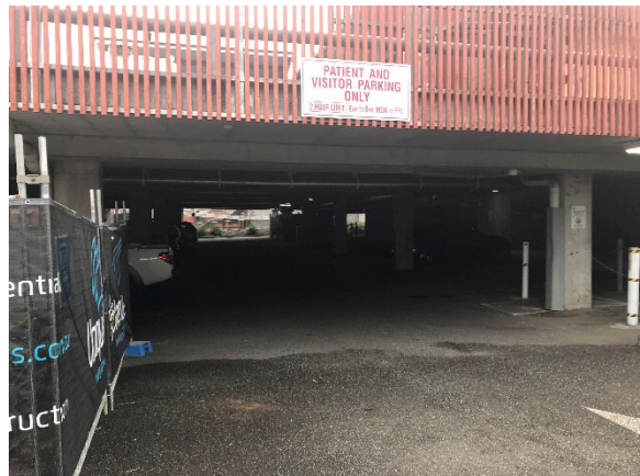
Plate 6.6 View north-west showing below-ground carpark in SU2 along High Street
