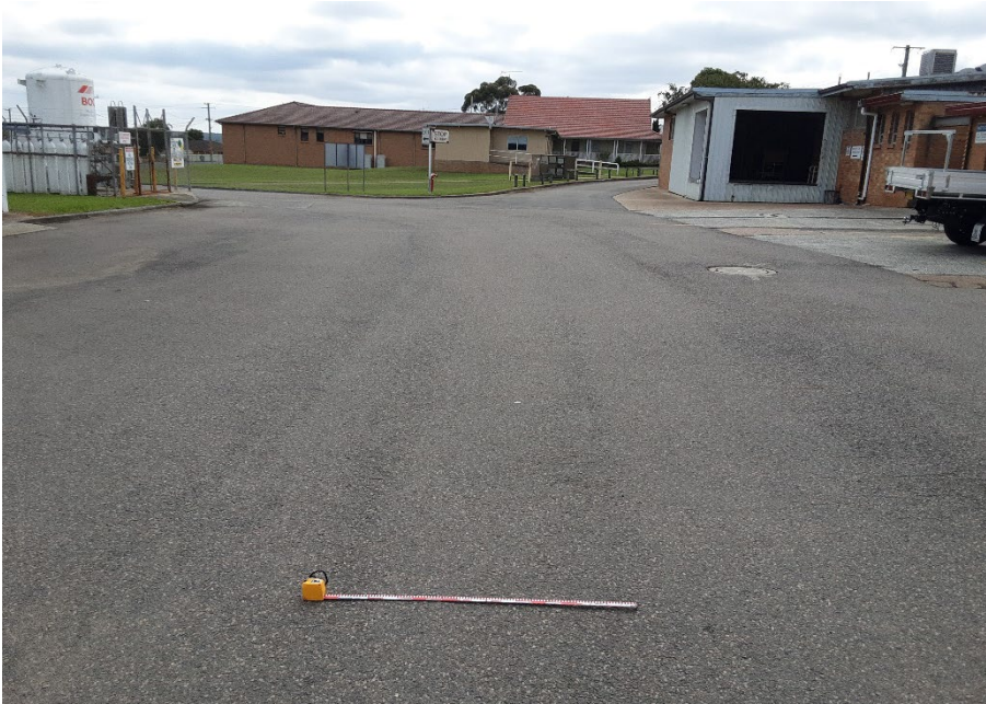
Photo 15 Tarmac driveway in the southern portion of the study area, facing east
