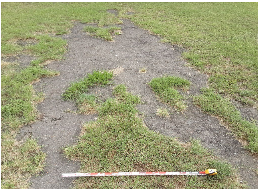
Photo 11 Exposure within the northern portion of the study area, facing north-west
