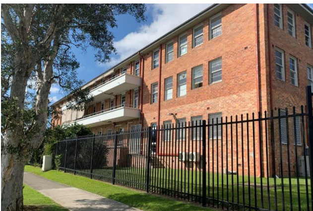
Plate 4.6 South-west elevation of Building 09 incl. concrete balconies.
