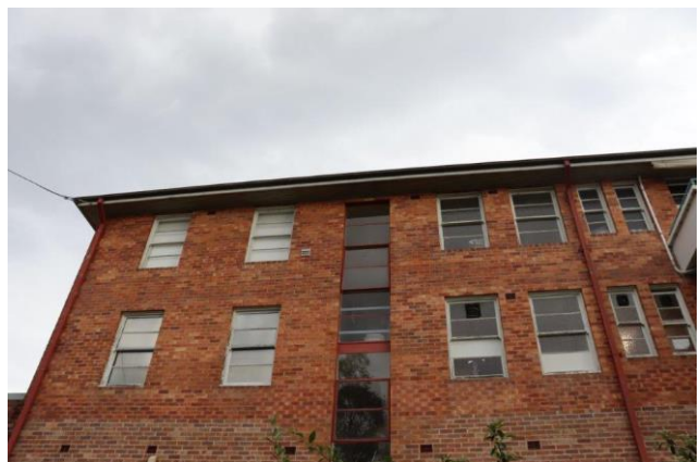
Plate 4.7 South-west elevation of Building 09.
