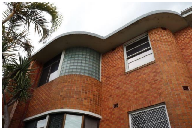
Plate 4.3 External window and roof detailing to Building 09 c.1941 structure.
