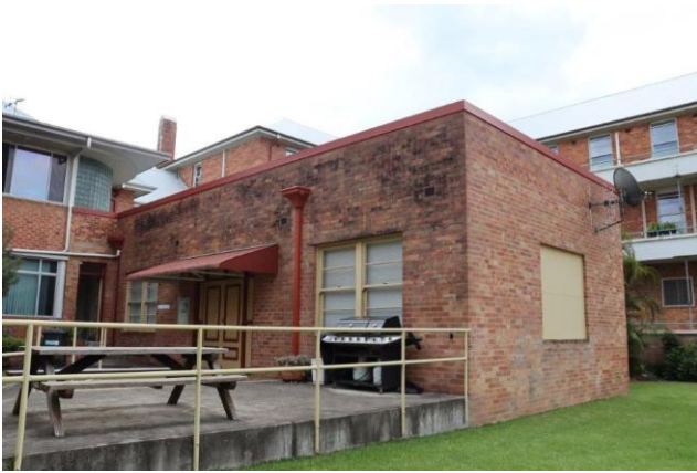
Plate 4.4 Single storey c.1954 extension to south-east elevation of Building 09.
