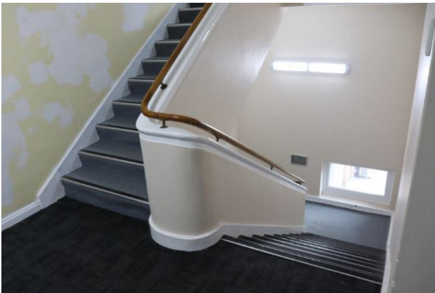
Plate 4.12 Stairway to c.1954 section of Building 09.
