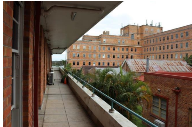
Plate 4.13 Concrete balconies to c.1954 section of Building 09.
