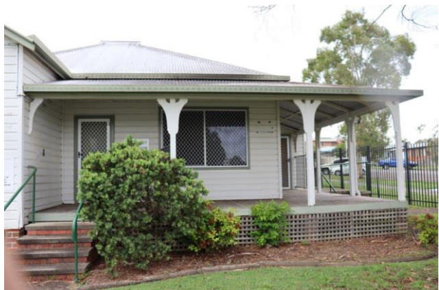
Plate 4.17 North east elevation and verandah to Building 11.
