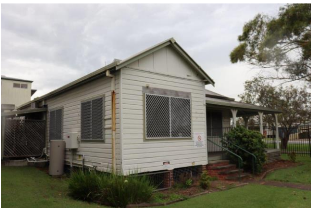
Plate 4.16 North-east elevation of Building 11.
