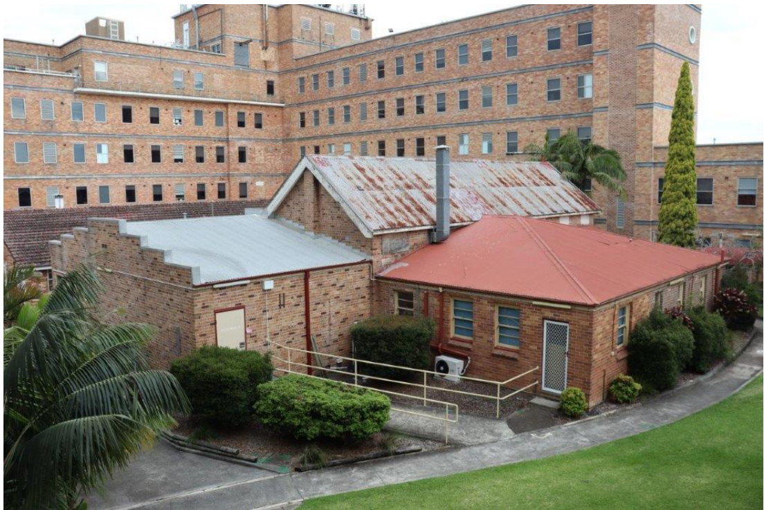
Plate 3.14 Photograph of the Victoria Fever Ward. Source: EMM 2021
