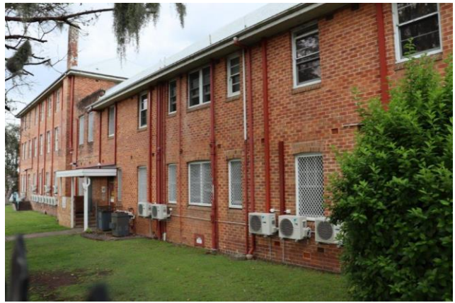
Plate 4.5 Transition from c.1941 to c.1954 structure to south-west elevation of Building 09.
