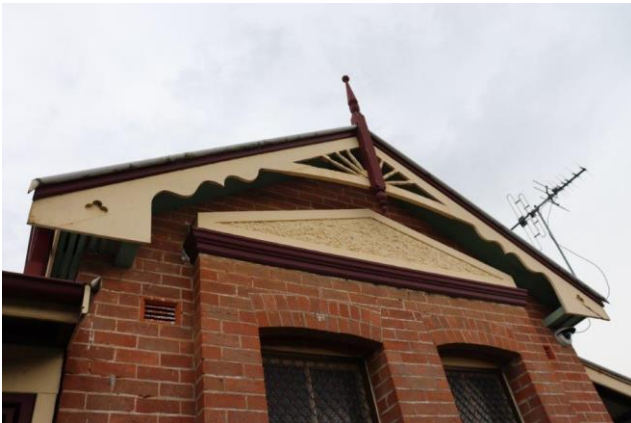
Plate 4.14 Roof structure, gable and upper section to south-east elevation of Building 11.
