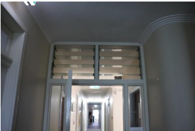
Plate 4.10 Curved wall section and glazed doorway with louvred fanlight, to Building 09 upper level.
