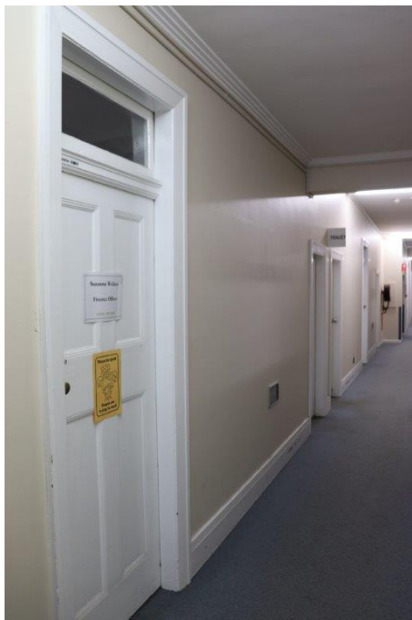
Plate 4.8 Remaining c.1921 walls and door openings to Building 09.
