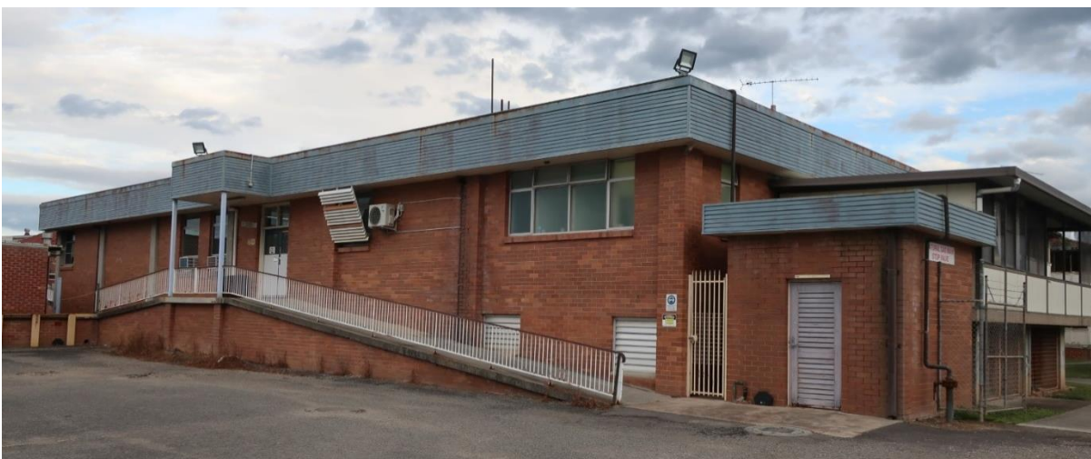
Photo 3.9 East view towards the rear of Building 8, facing the car park
