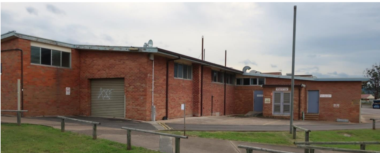
Photo 3.11 The eastern industrial Building 9 from the c1950s would be demolished
