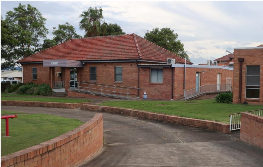
Photo 3.6 Building 4 was built in the 1930s
