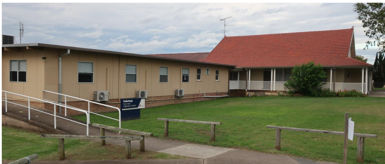
Photo 3.16 The c1960s Building 12 on the left would be removed, and the Federation Building 13 on the right would be retained
