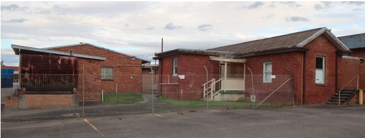
Photo 3.12 The service buildings that are Building 11. The building on the right is likely from the 1920s. The post war building on the left would be demolished.
