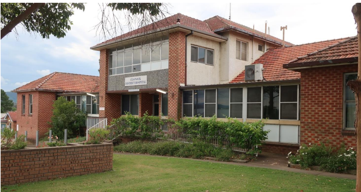
Photo 3.7 The altered front section of the Drinkwater Building (Building 5) facing View Street
