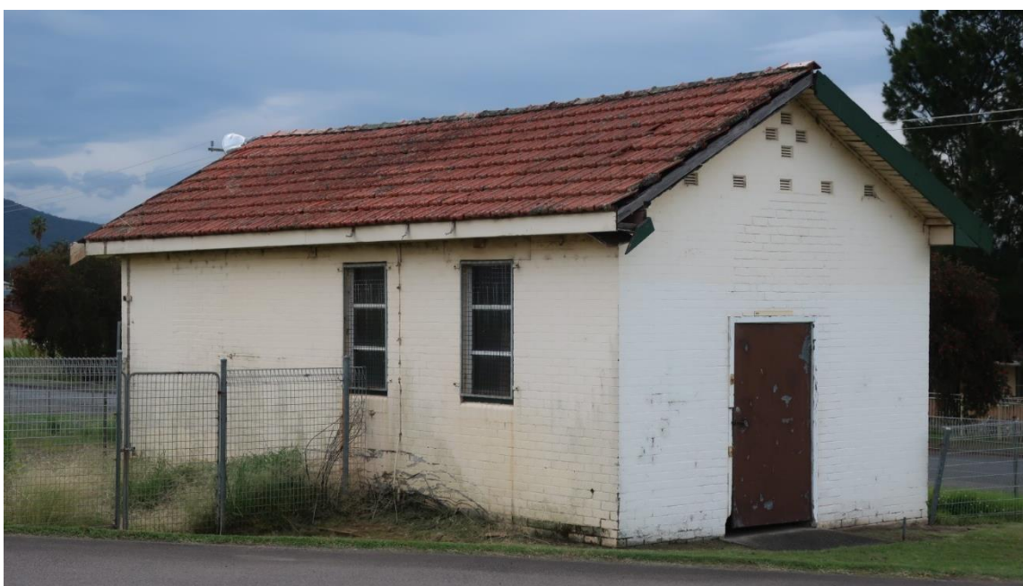
Photo 3.19 The inter-war mortuary Building 14 would be demolished
