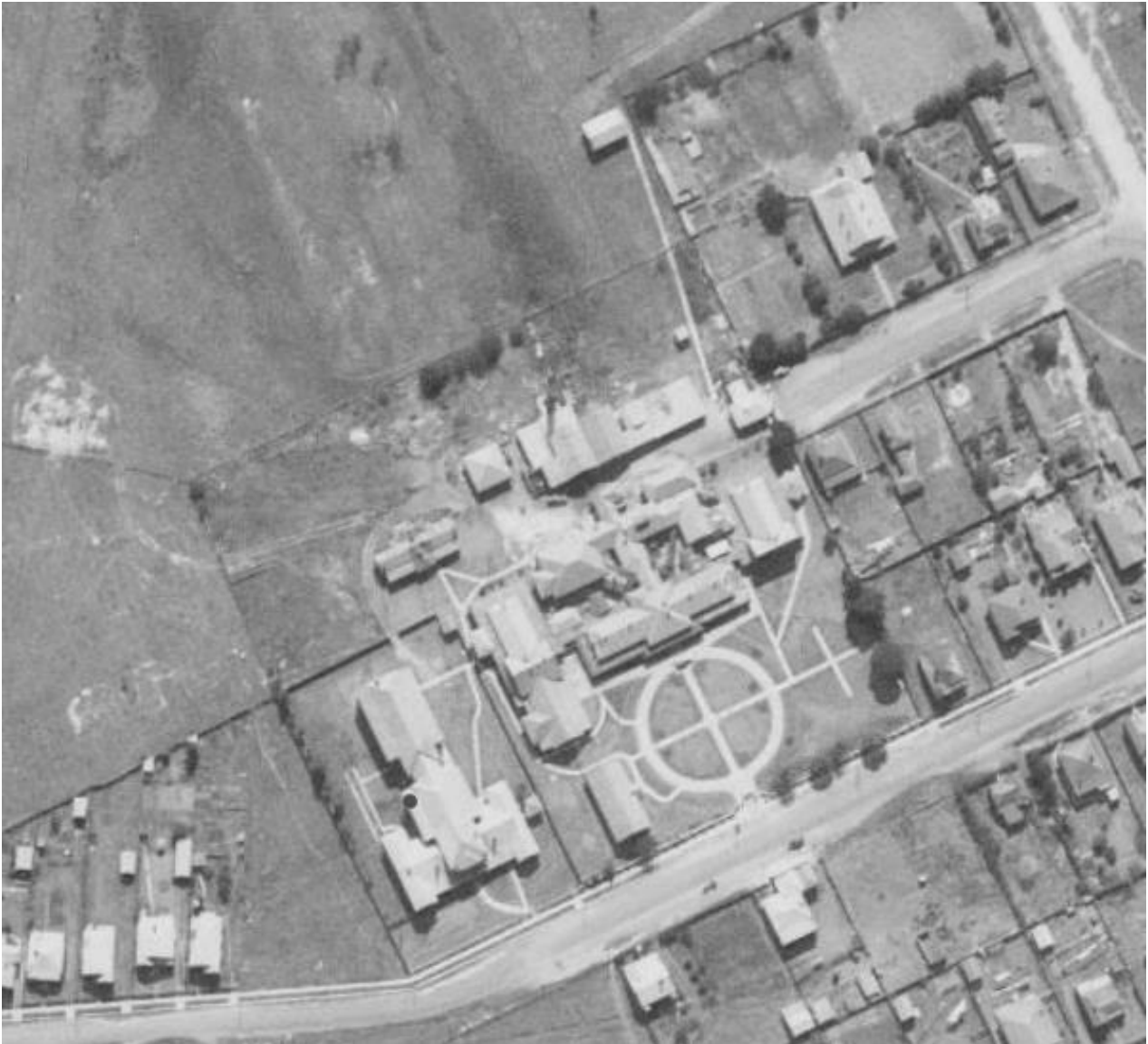
Figure 2.6 1944 aerial photograph of the Cessnock Hospital.
