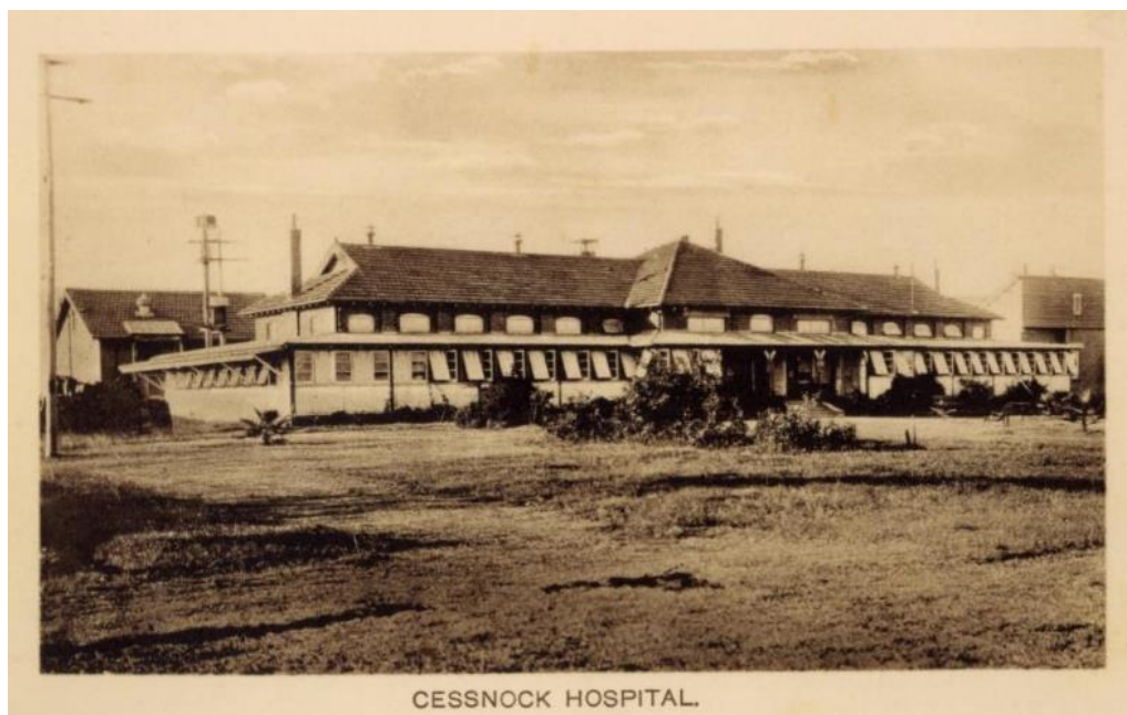
Figure 2.3 Cessnock Hospital c1930, looking north-east, showing verandah infilled and the operating theatre on the far left
