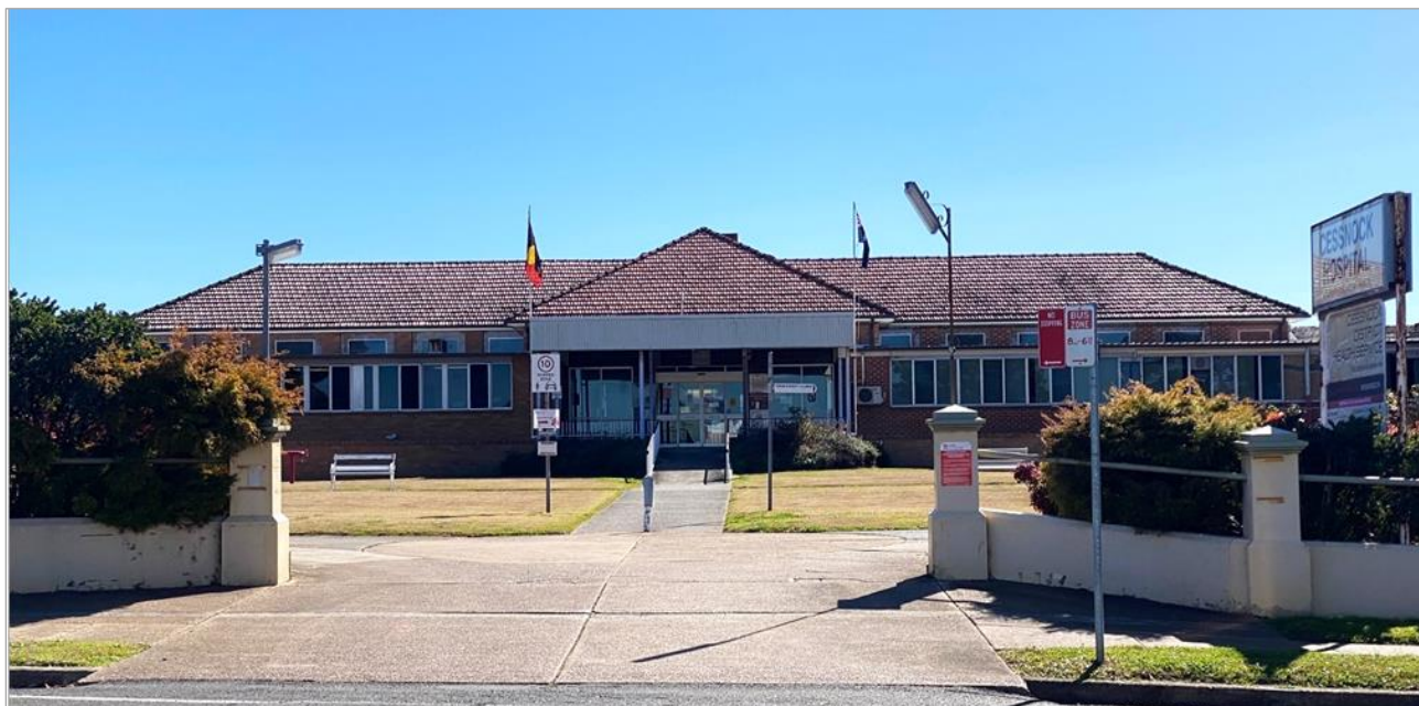
Cessnock Hospital: 24 View Street, Cessnock NSW 2325
