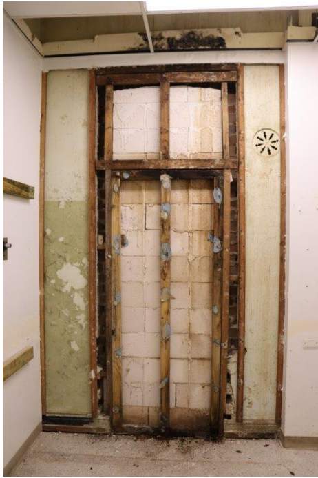
Plate 4.24 Exposed section of original north-west wall and former door opening.
