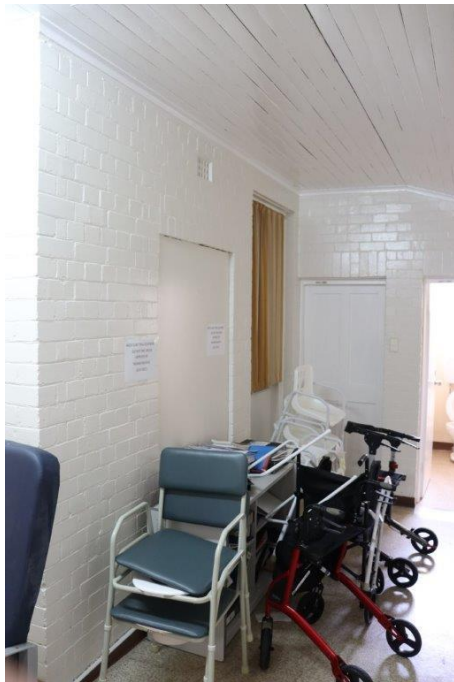
Plate 4.14 Interior space c.1932 extension to south-west.
