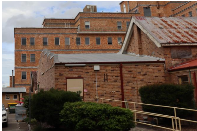
Plate 4.7 c.1990 extension to the north-west elevation of the original building.
