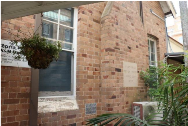
Plate 4.10 Exposed original south-east elevation.
