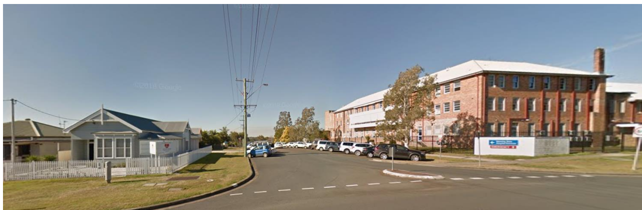
Plate 7.2 Small weatherboard cottage along York Street (I128 GTLEP) (left) in relation to hospital site and existing Building 09 (right). Source: Google Maps 2017.
