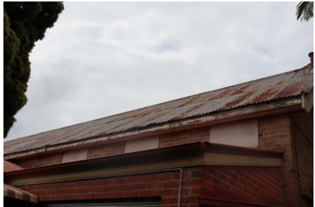
Plate 4.9 Roof and upper section of original building to south-west.
