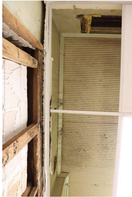
Plate 4.25 Exposed original ceiling incl. corrugated ceiling and cornice.
