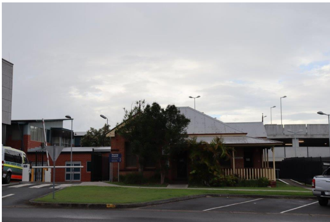
Plate 3.28 Brick cottage (I154 GTLEP) as seen along High Street. Source: EMM 2021
