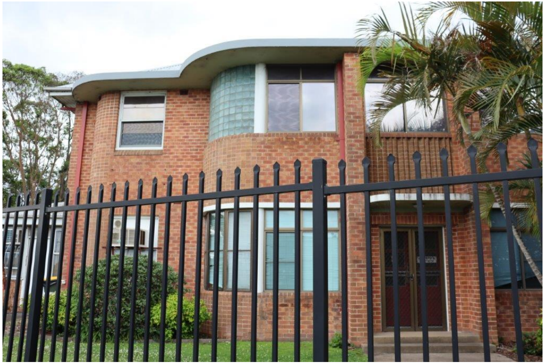
Plate 3.17 South-east elevation to c.1941 nurse's quarters building section. Source: EMM 2021
