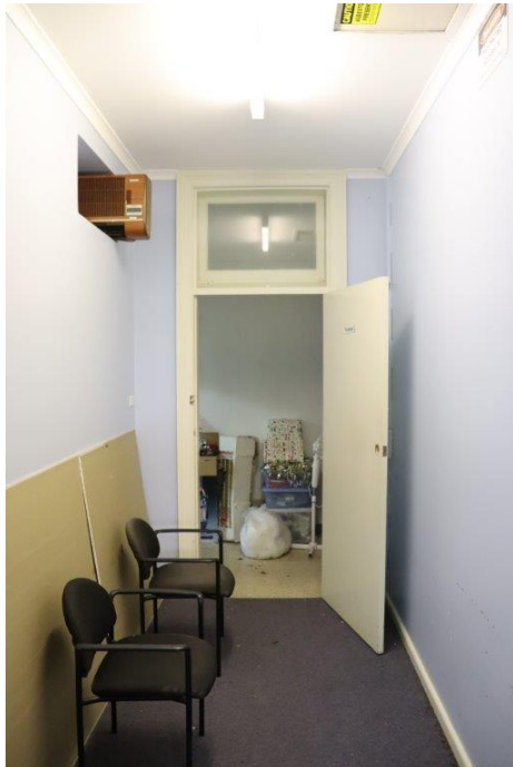
Plate 4.20 Original door opening and fanlight to hallway.
