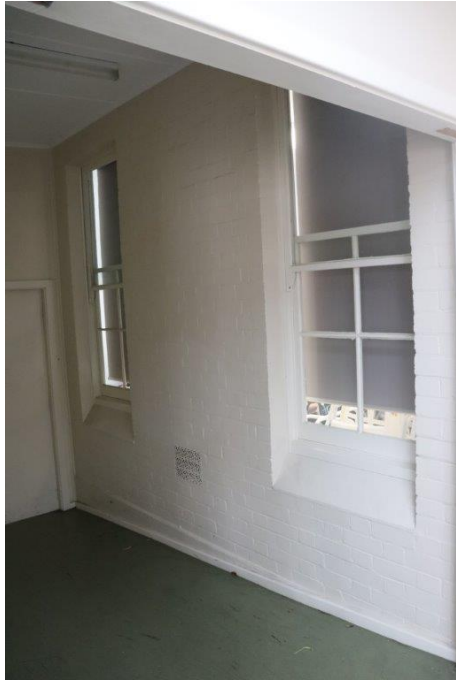
Plate 4.18 Exposed original north-east elevation with original timber windows.
