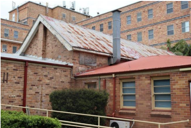
Plate 4.8 Roof and upper section of original building to north-west.
