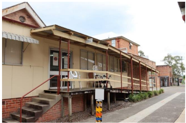
Plate 4.5 c.1967 extension to north-east elevation of original building.
