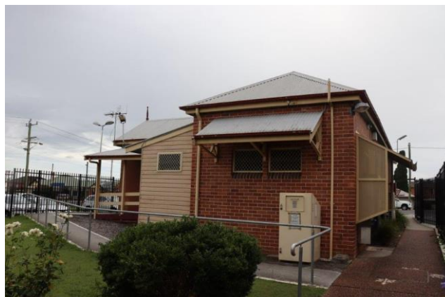
Plate 2.2 Later addition and rear section of Building 11.
