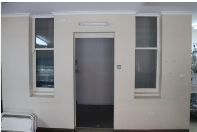
Plate 4.16 Original Fever Ward main entry with timber framed windows.
