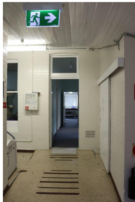
Plate 4.23 Original door opening and window to enclosed south-west elevation.
