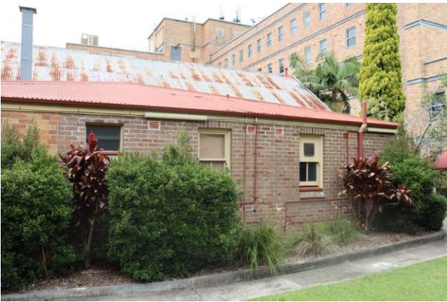
Plate 4.2 c.1934 and .1950s extension to the south-west of the original building.
