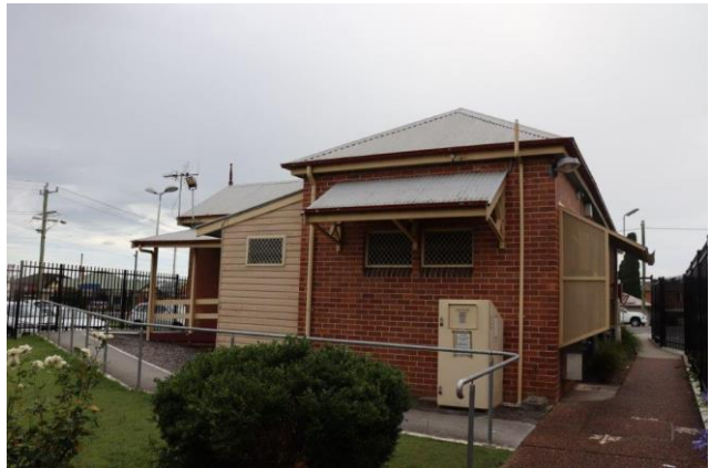
Plate 4.27 Later addition and rear section of Building 11.
