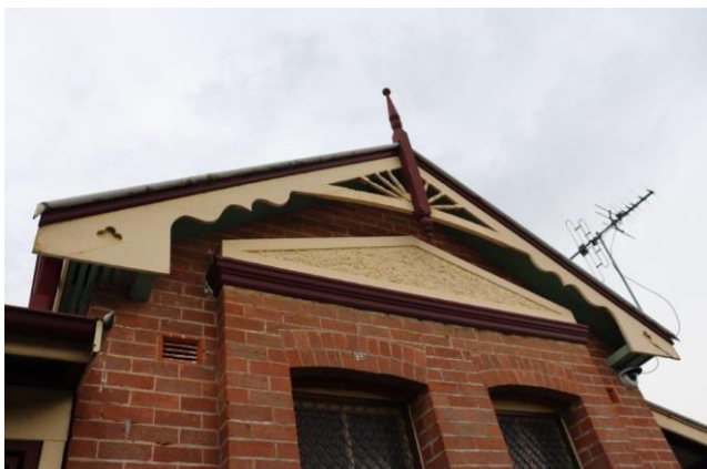
Plate 2.1 Roof structure, gable and upper section to south-east elevation of Building 11.
