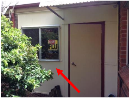
Photo No. 004: Southern elevation (outside Room MN0800008)
