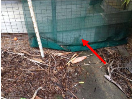
Photo No. 001: Below south entrance ramp
