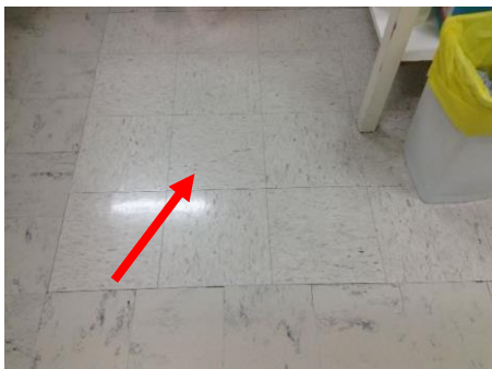
Photo No. 012: Ground Floor MN0700015
