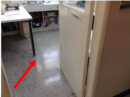
Photo No. 010: Ground Floor MN0700007 (Microbiology)
