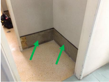
Photo No. 024: Ground Floor MN0700002
