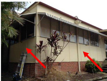
Photo No. 003: South-east extension
