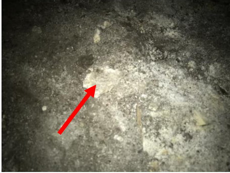
Photo No. 018: Subfloor
