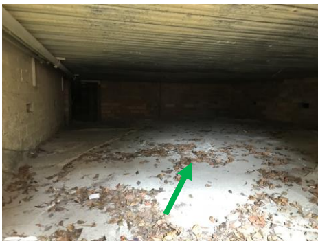
Photo No. 026: Subfloor
