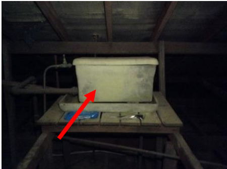
Photo No. 005: Ceiling Void
