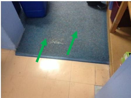
Photo No. 026: Ground Floor (MN0700023)
