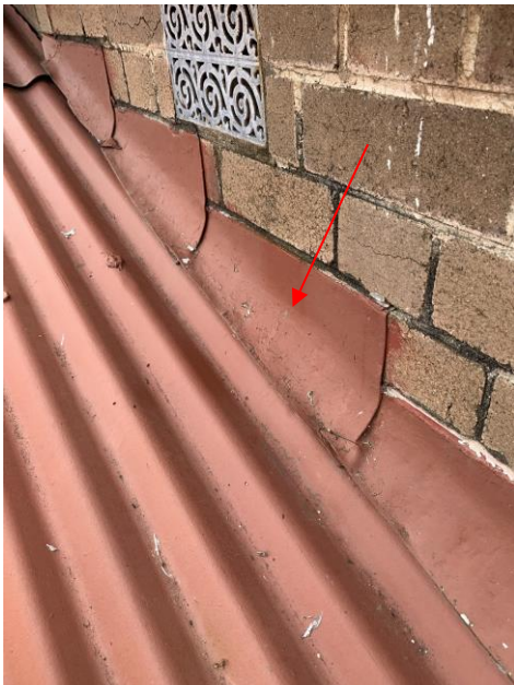
Lead: Flashing
