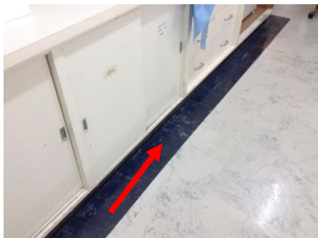
Photo No. 011: Ground Floor MN0700015
