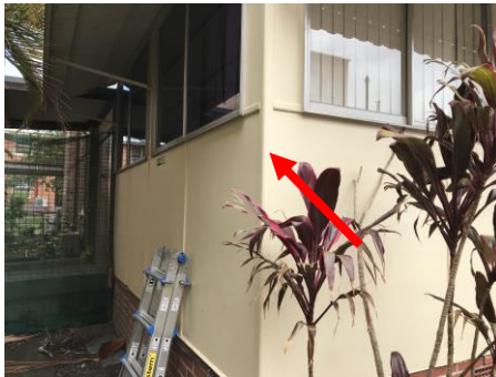
Photo No. 002: South-east extension
