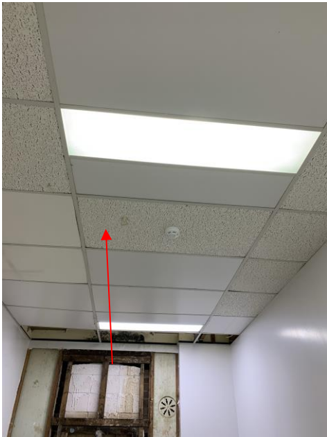
SMF: Ceiling tiles
