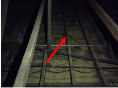
Photo No. 004: Ceiling Void
