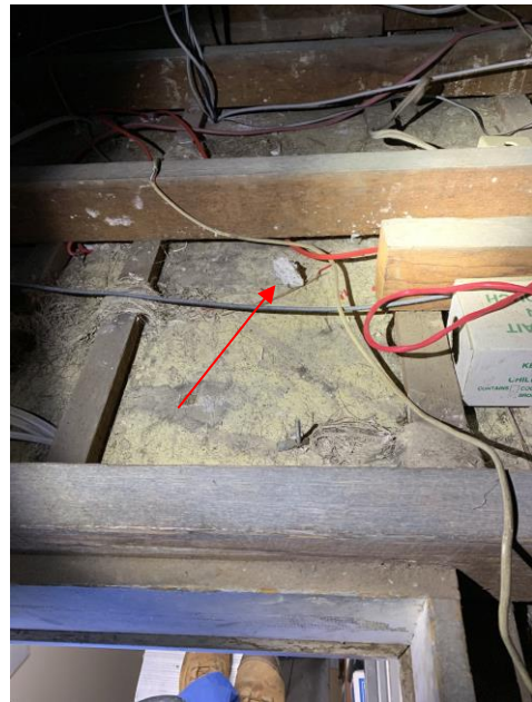
AS14 – 10: Chrysotile, Amosite and Crocidolite asbestos
