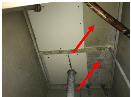
Photo No. 006: Ceiling Void (Above Storage Room)
