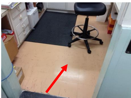
Photo No. 015: Ground Floor tiled area in MN0700018
