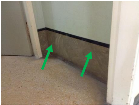
Photo No. 025: Ground Floor MN0700005 (Men's Shower and Toilet)
