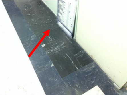
Photo No. 013: Ground Floor MN0700015
