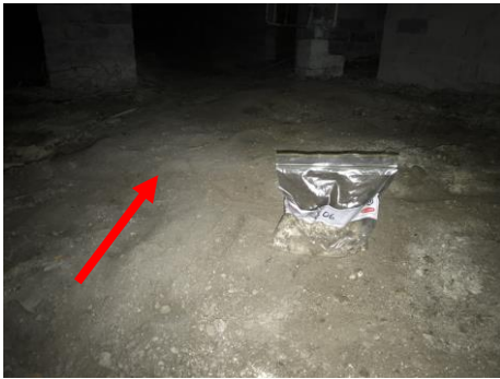
Photo No. 017: Subfloor
