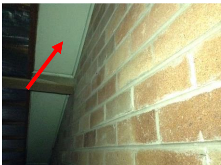
Photo No. 009: Ground Floor ceiling void above MN0700007
