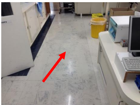
Photo No. 014: Ground Floor MN0700015
