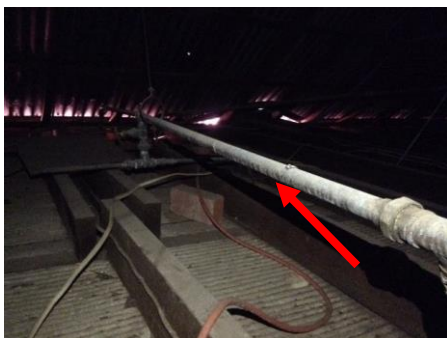
Photo No. 006: Ceiling void MN0800006
