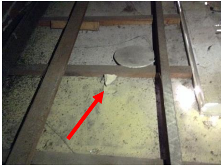
Photo No. 007: Ceiling Void (MN070007)
