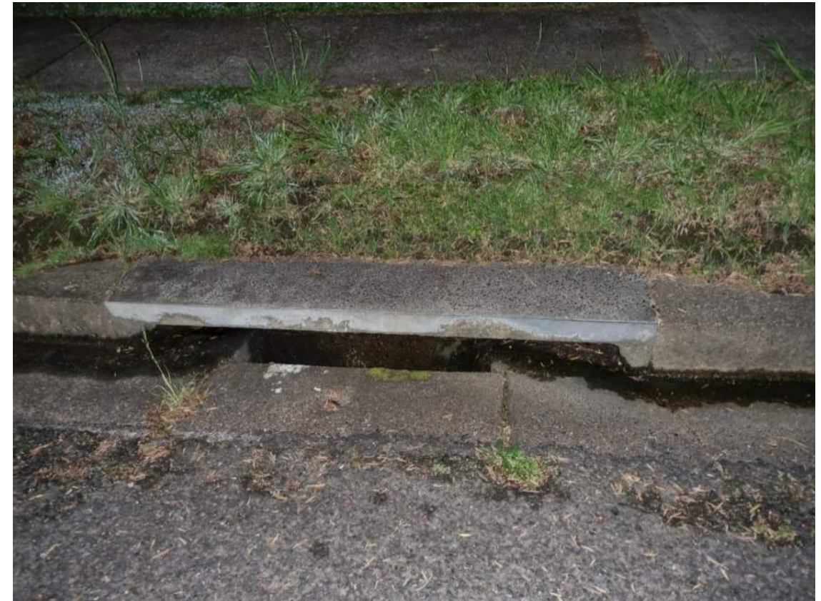
Figure 9: Existing Council Sag Pit on View Street
