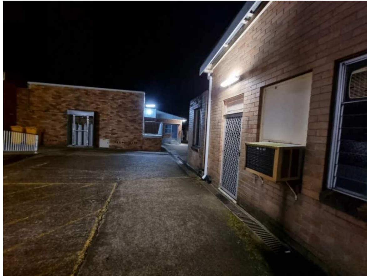
Figure 7: Downpipe Discharging into Grated Drain
