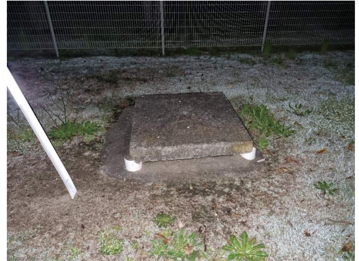
Figure 8: Existing Council Letterbox Pit on Jurd Street
