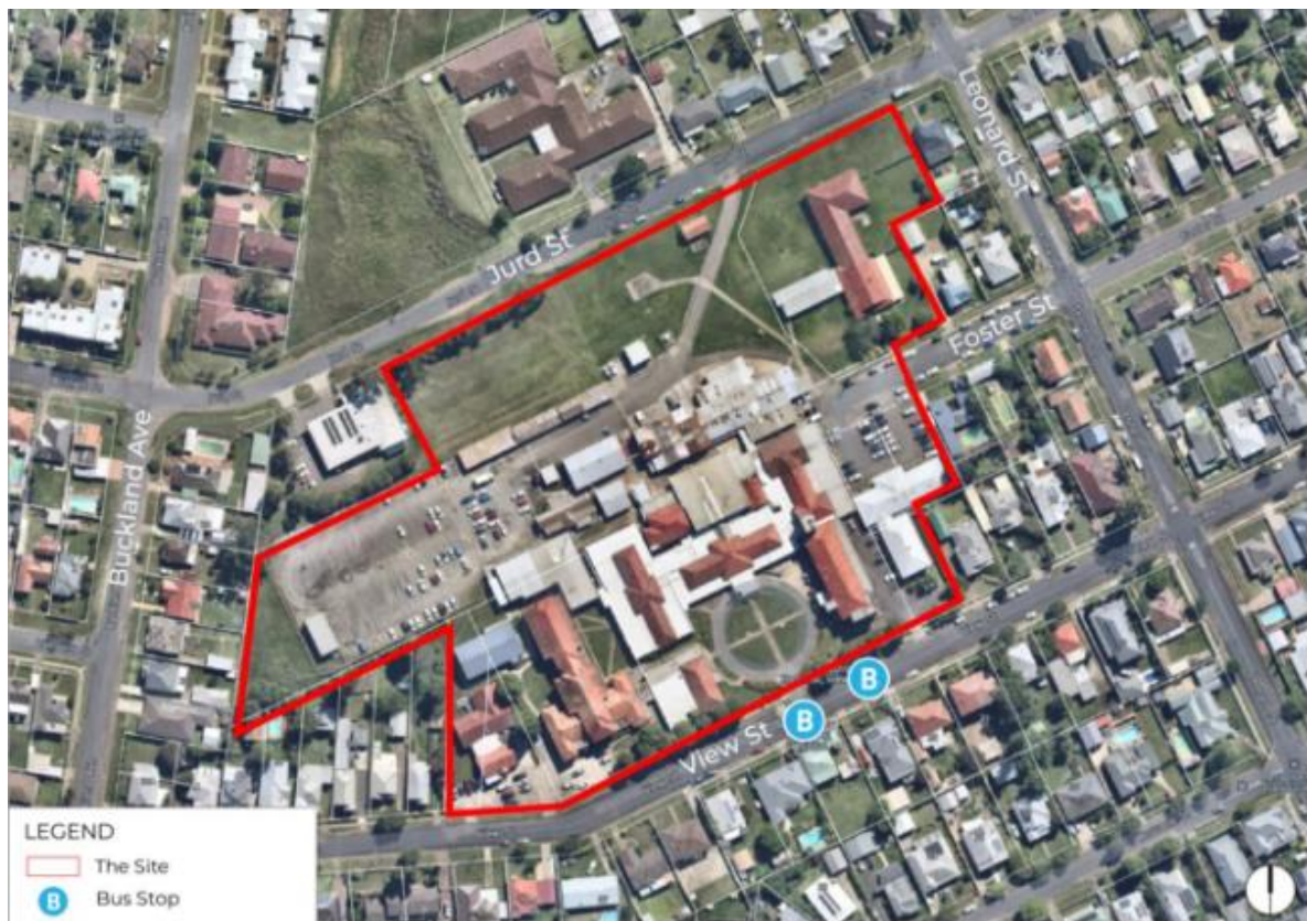
Figure 1: Aerial view showing the Cessnock Hospital site (Source: Nearmap).
