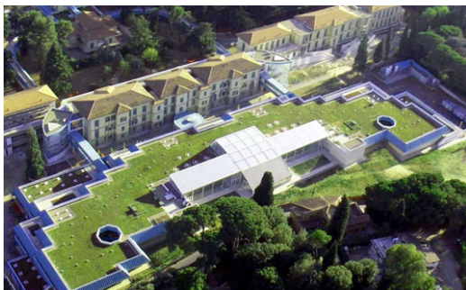
Figure 7 Meyers Paediatric Hospital, Florence, Italy. Green Roofs provide flood control plus therapeutic benefits
