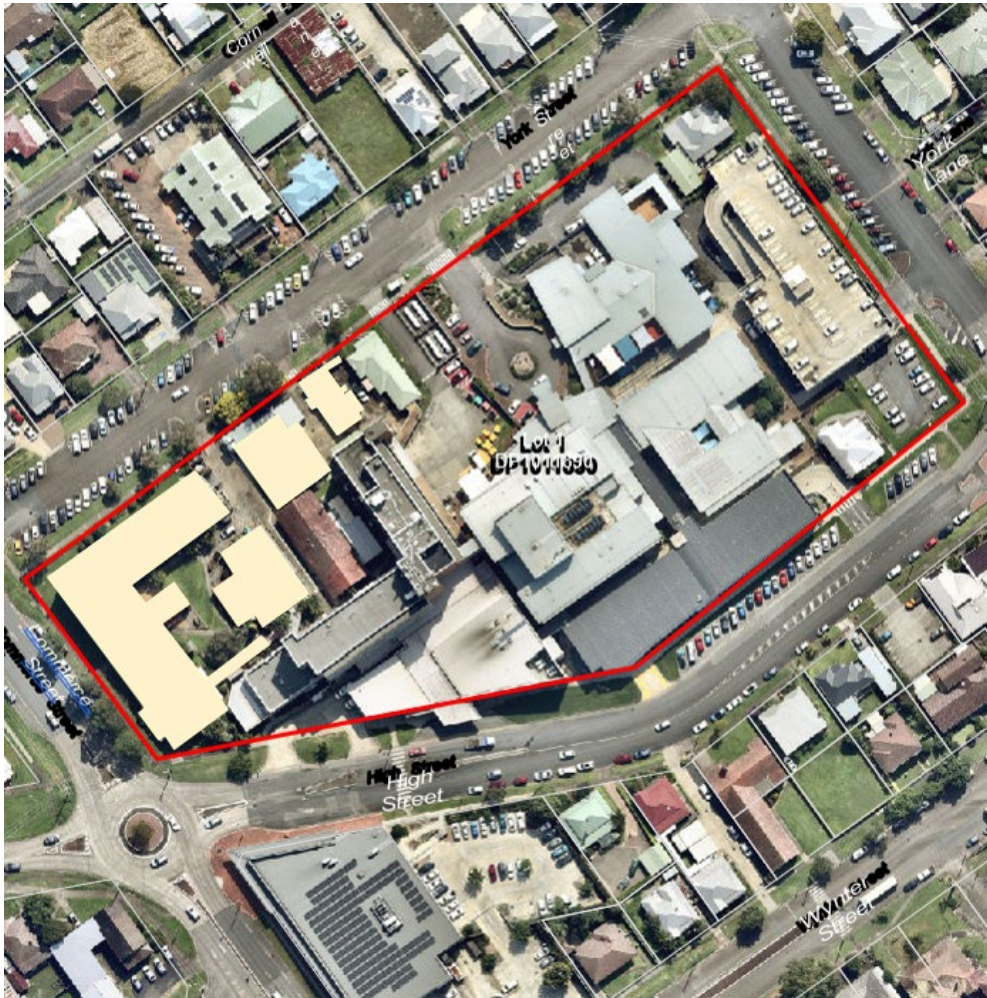
Figure 2 - Aerial photo showing the buildings within the hospital site boundaries in red. The four buildings highlighted in beige are proposed to be demolished.
