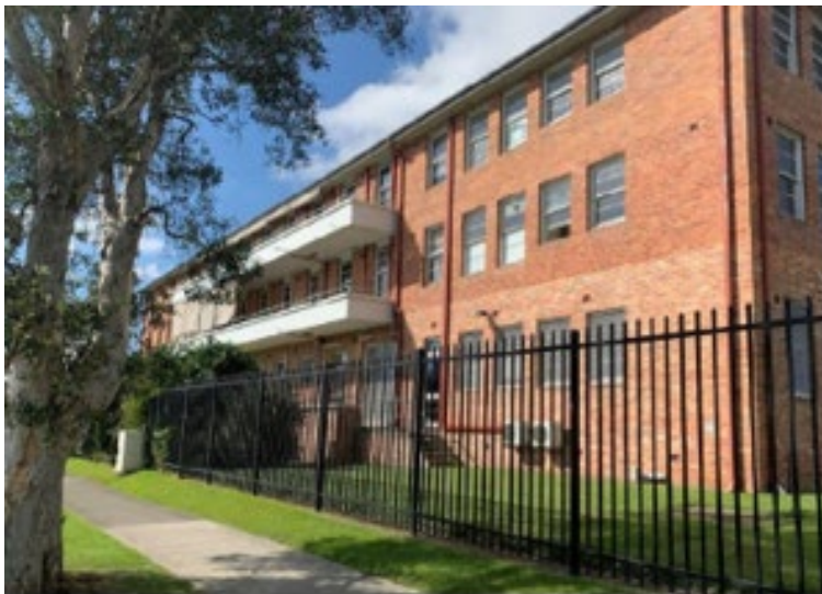
Photo 2: South-east elevation of Building 9 (Administration/Nurses Quarters)
