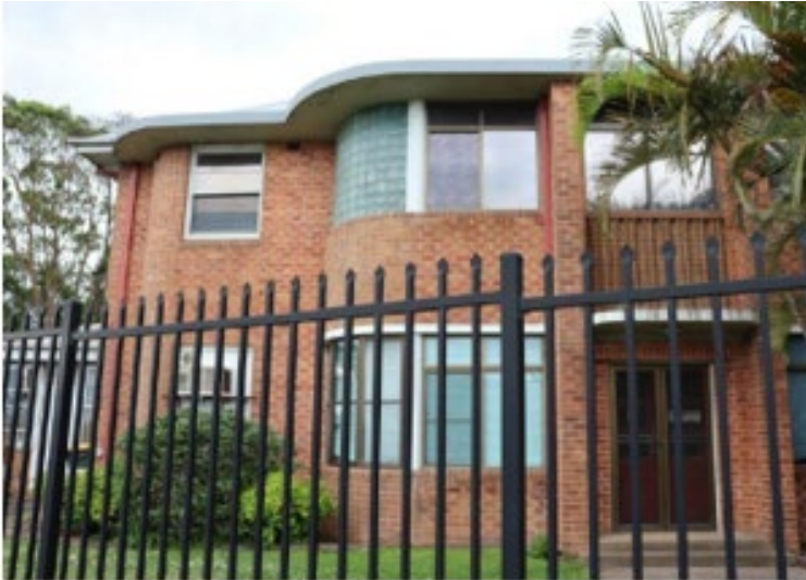
Photo 1: South-east elevation of Building 9 (Administration/Nurses Quarters)
