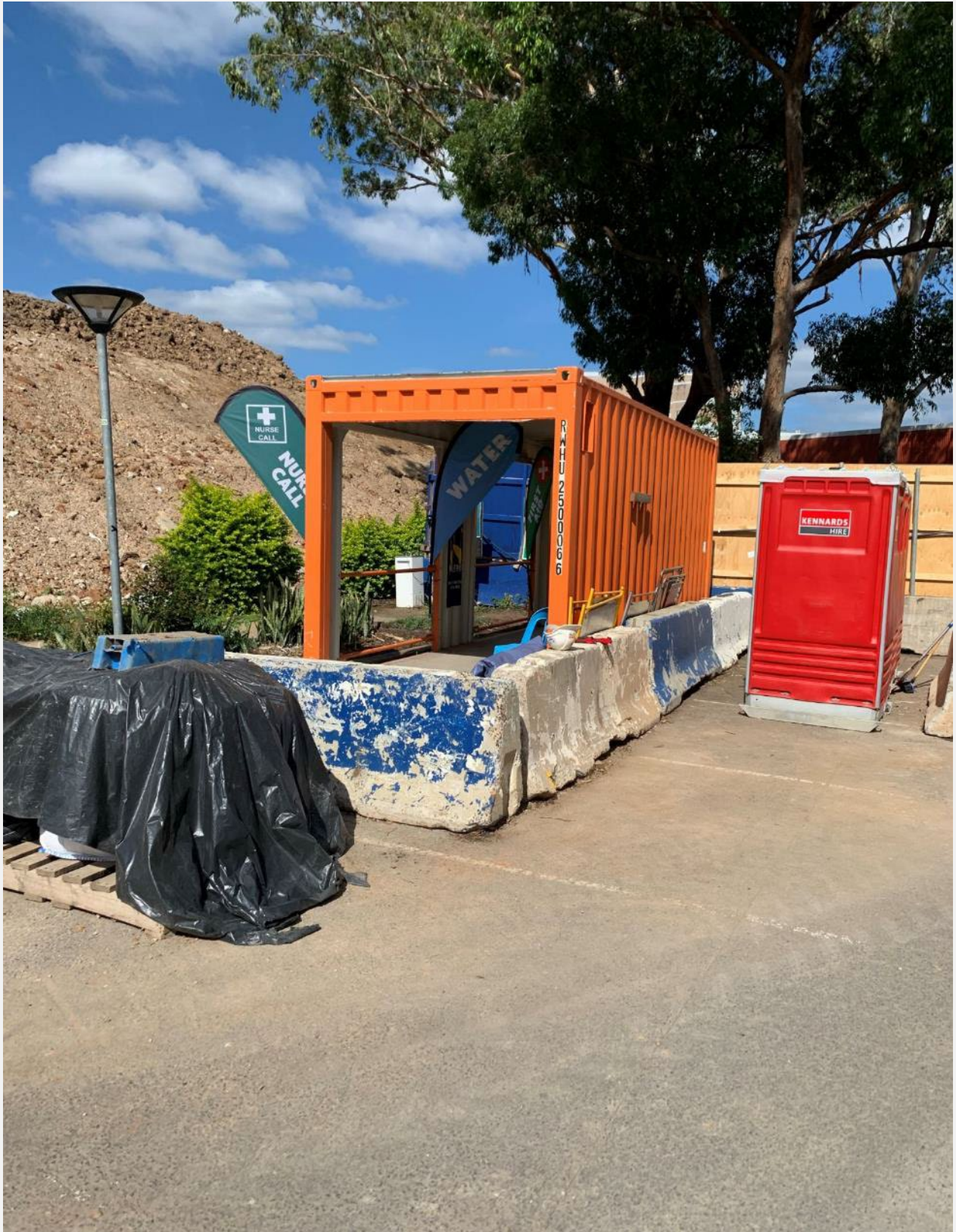
Photo 22 – Water stand, safety station and amenities available on site
