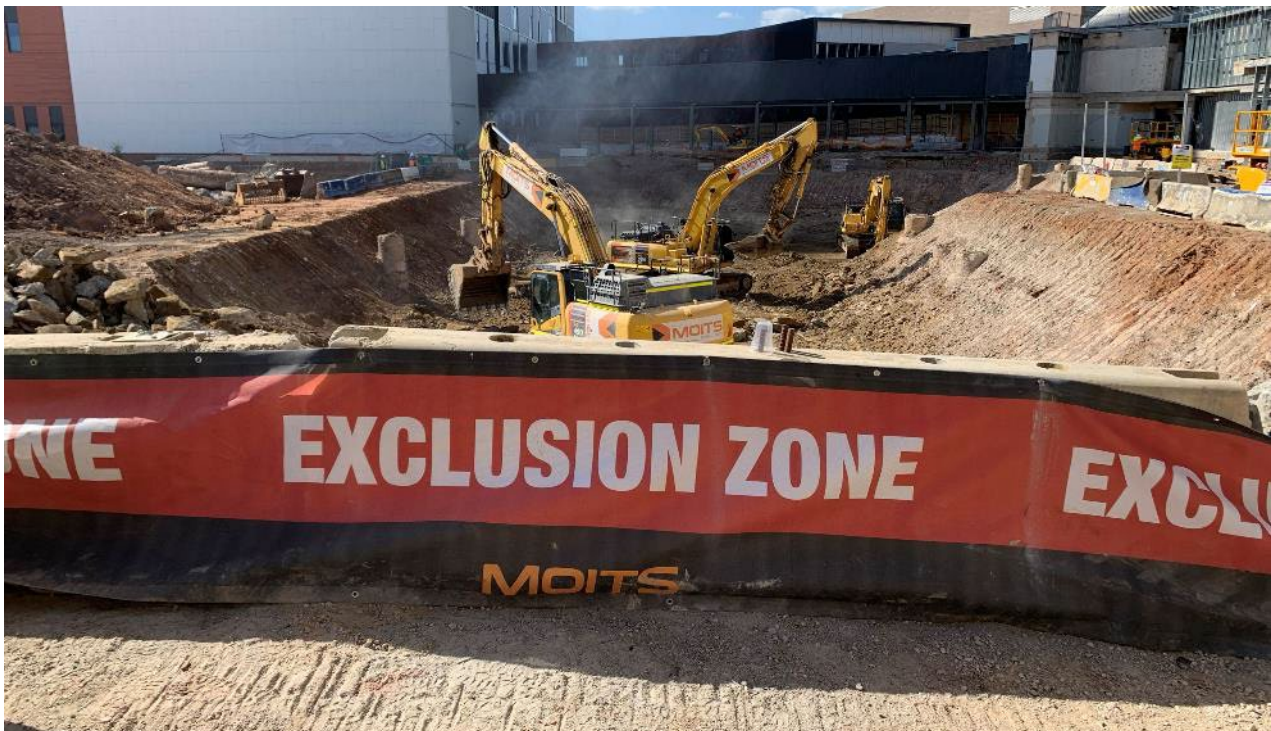
Photo 13 – Exclusion Zone barriers in place
