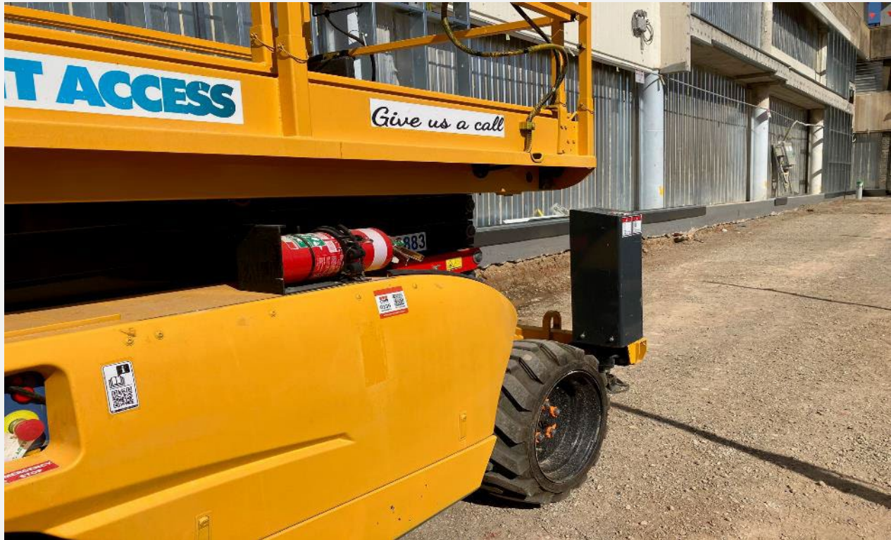
Photo 26 – Plant on site
