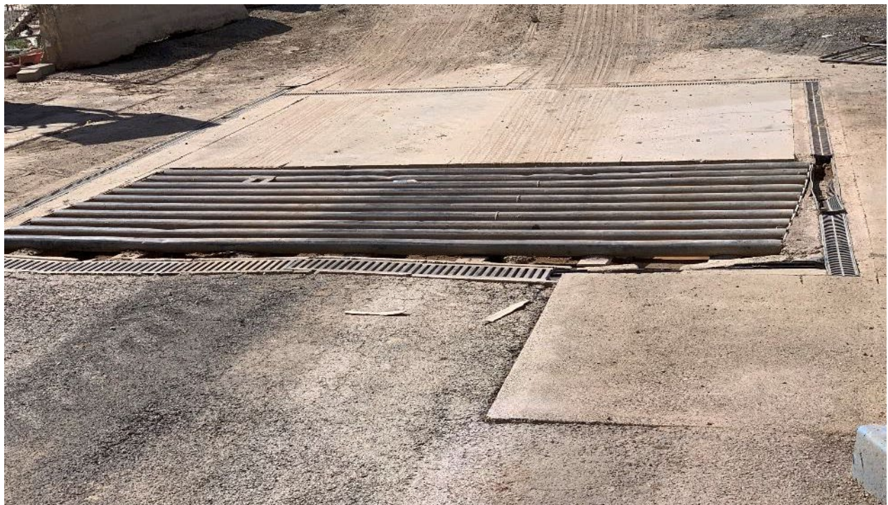
Photo 9 – Rumble grid and hard stand area installed at the site entrance
