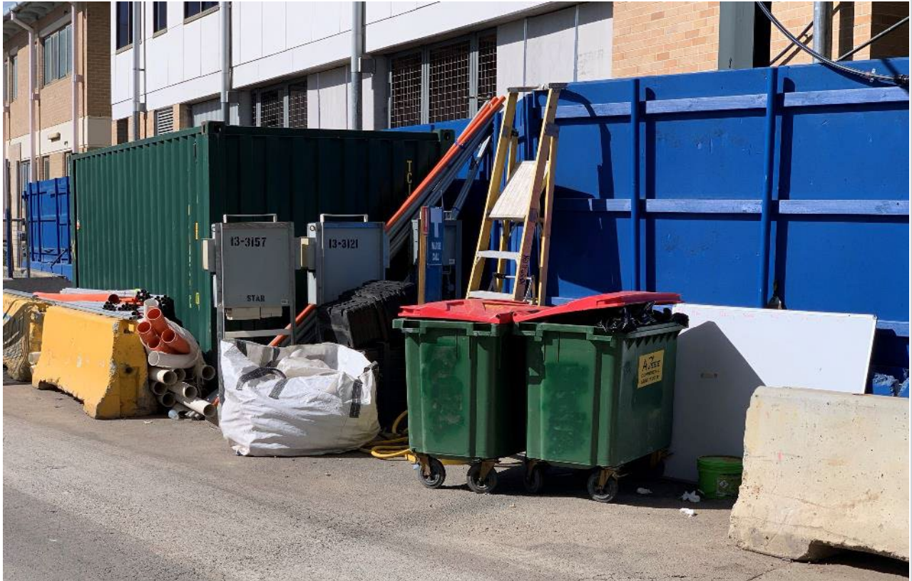
Photo 8 – Waste Bins available on Site
