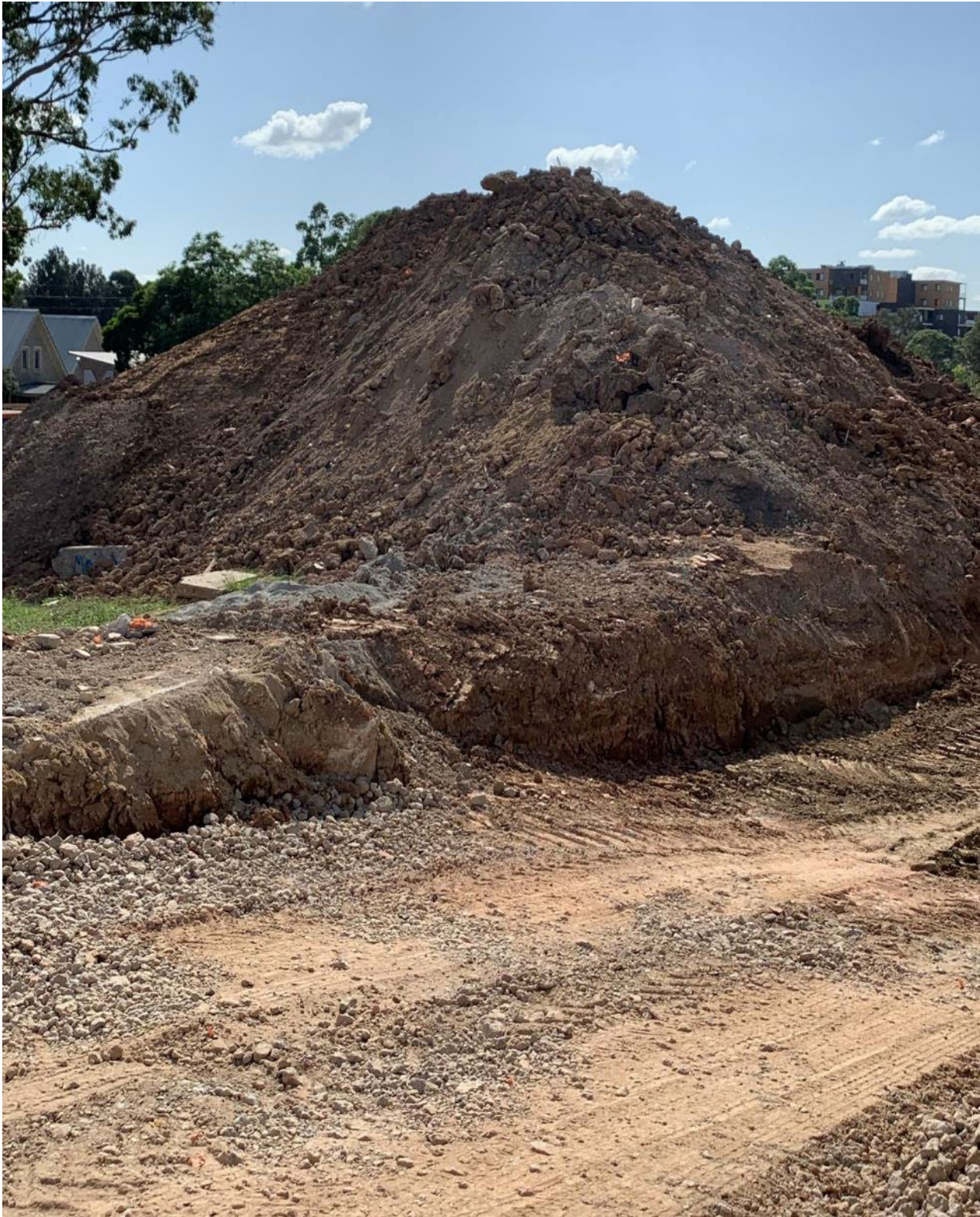
Photo 16 – Spoil from bulk excavation planned for later reuse onsite.
