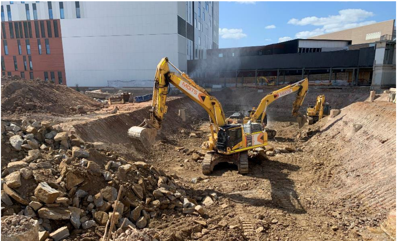
Photo 11 – Bulk Excavation in Progress
