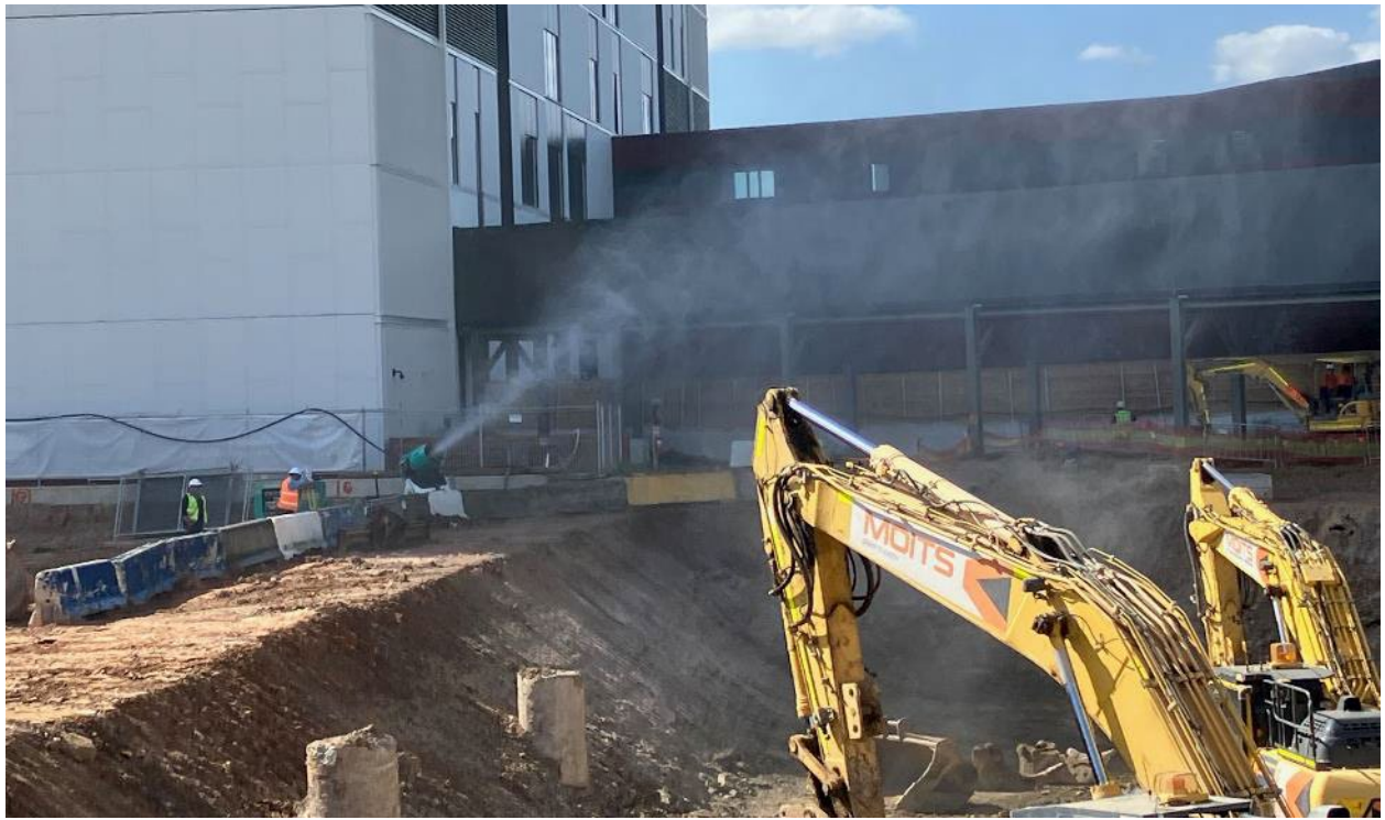
Photo 14 – Water Cannon in operation for dust suppression
