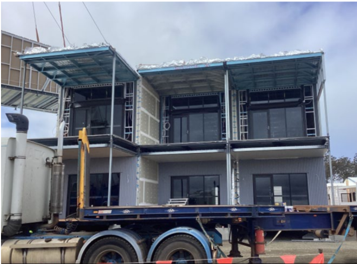
OFF-SITE MANUFACTURING OF THE KWA UNITS UNDERWAY (JULY 2024)
