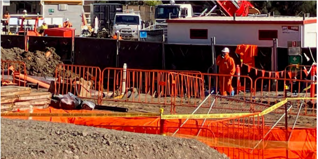
Workers observed in hazmat suits within asbestos exclusion zone.
