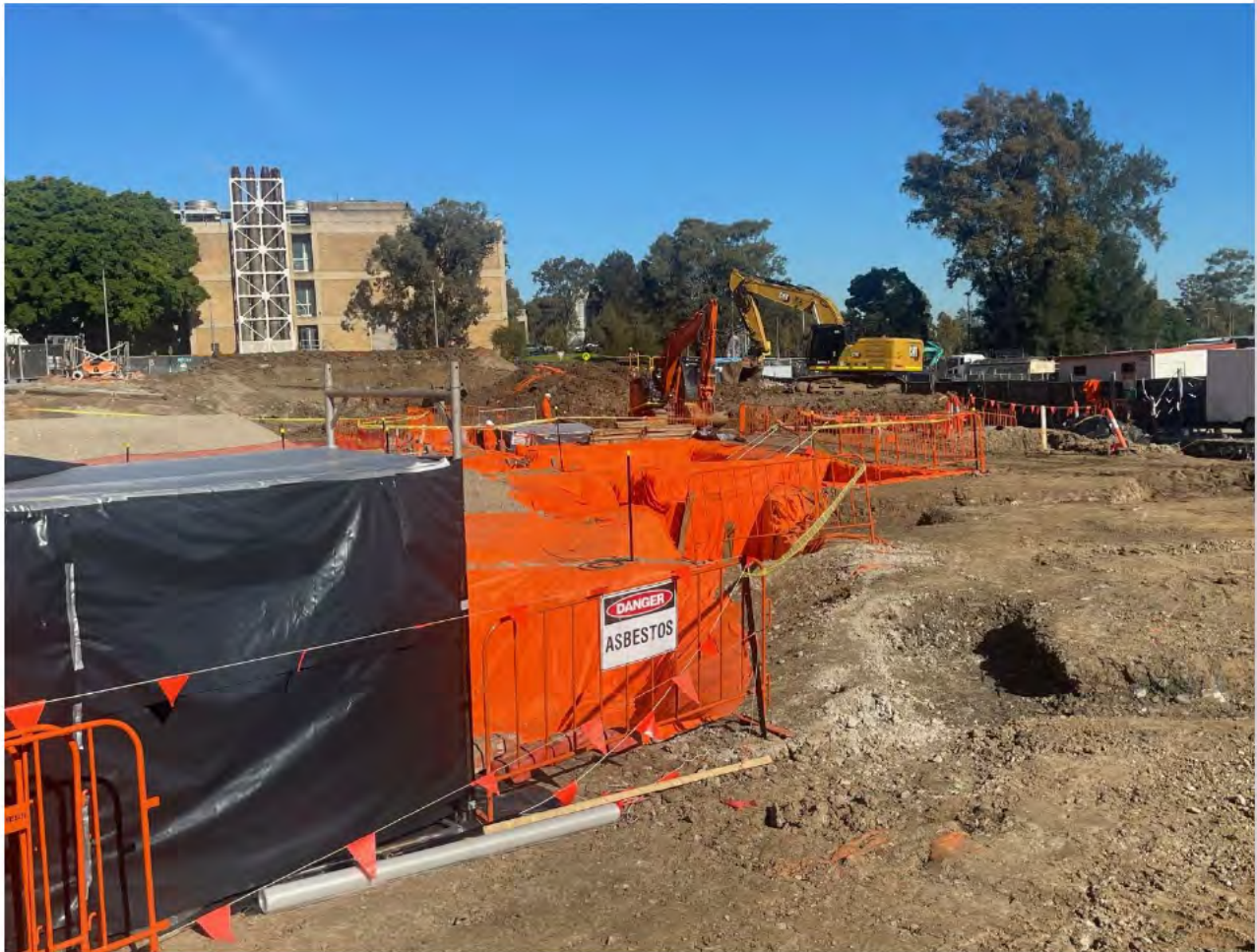
Orange geofabric being placed as a marker layer to identify residual contaminated material following backfill and capping.
