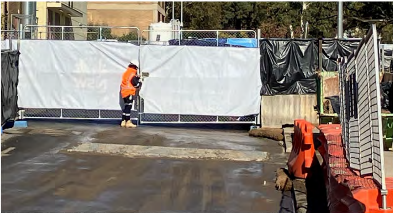
Gate secured when not in use.
