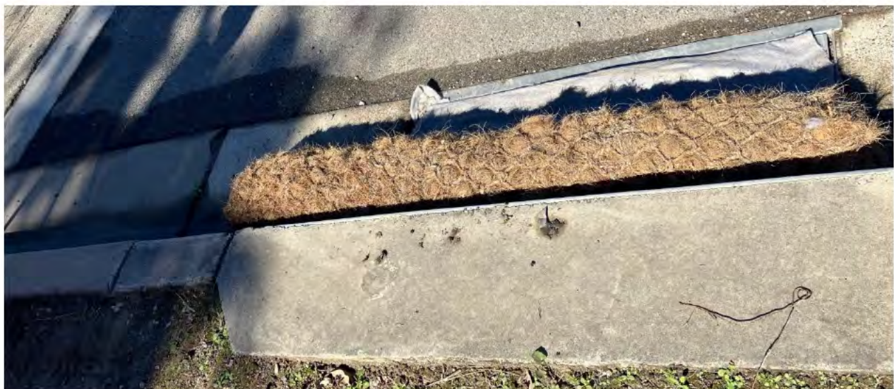
Protection of pit drain installed at Redbank Road during site inspection.
