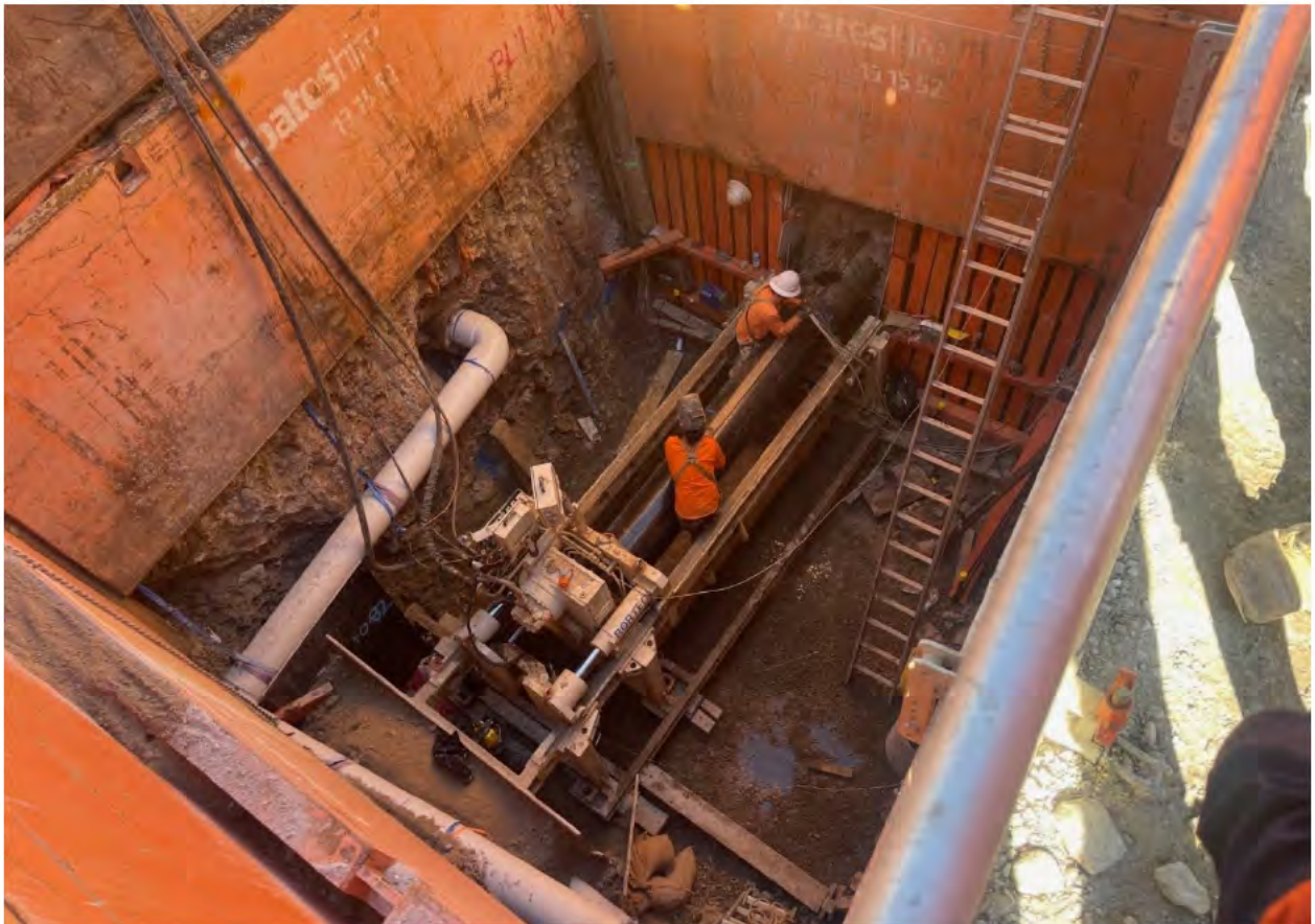
Horizontal drilling in uncontaminated material for services installation.
