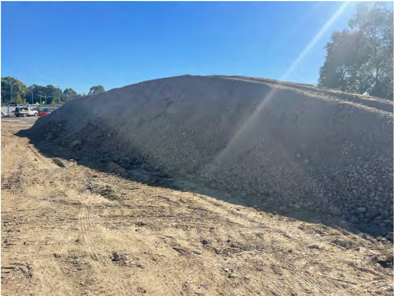
Stockpile noted to be quite steep in parts, however this is being progressively reused onsite
