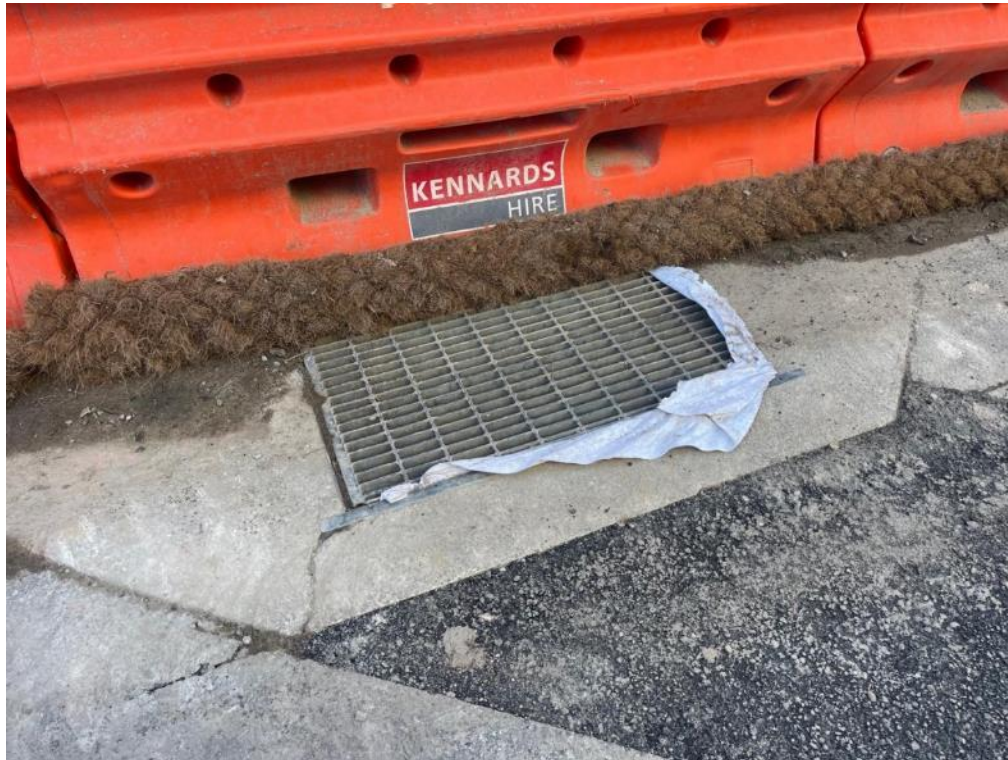
Pit drain protected with geofabric lining at Lambie Dew Drive.
