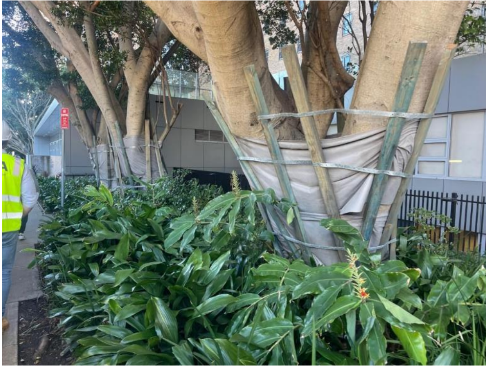
Tree protection in place adjacent to Temporary HLS.
