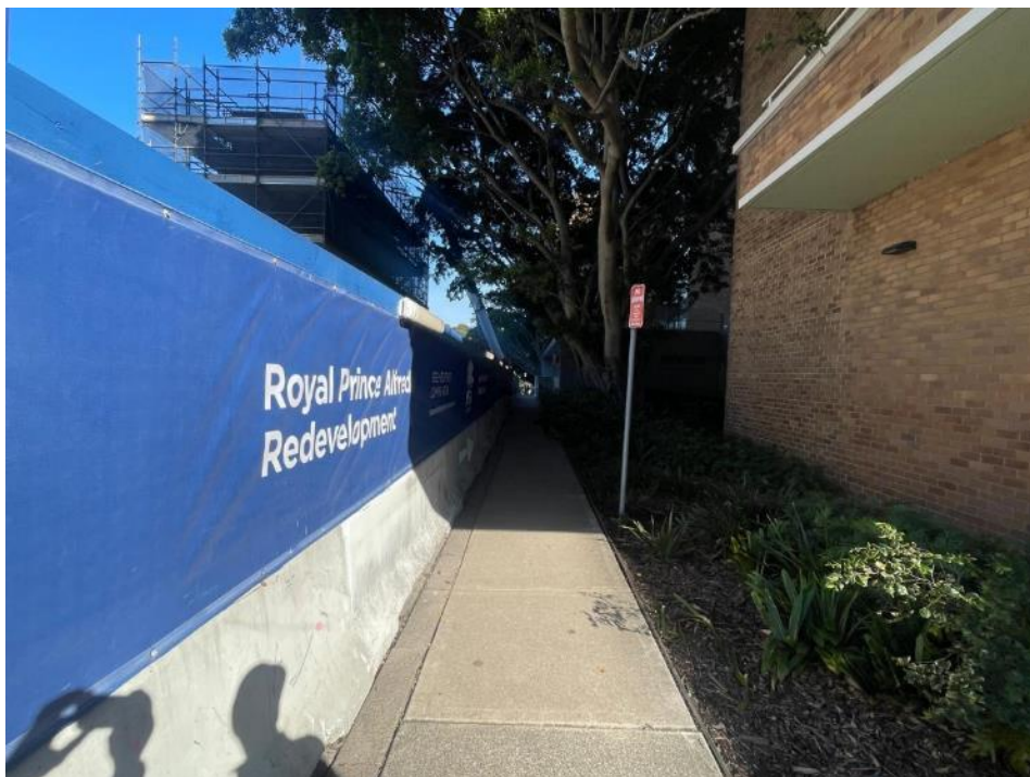
No obstruction of public way observed during the site inspection.
