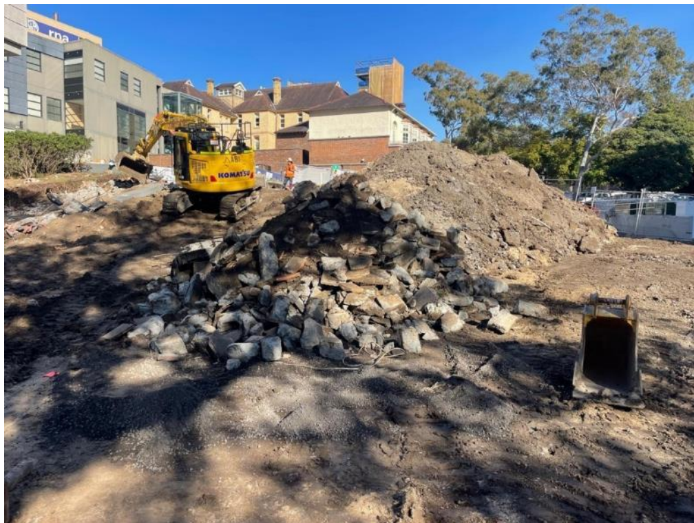
General Site construction activities were in progress. No dust observed.
