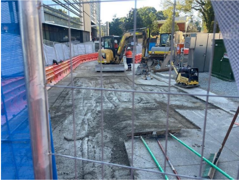
Johns Hopkins Drive entrance works in progress.
