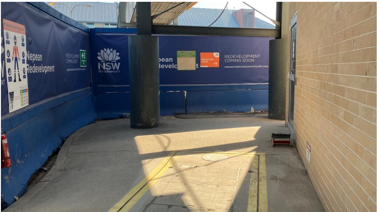
Hoarding and signage installed
