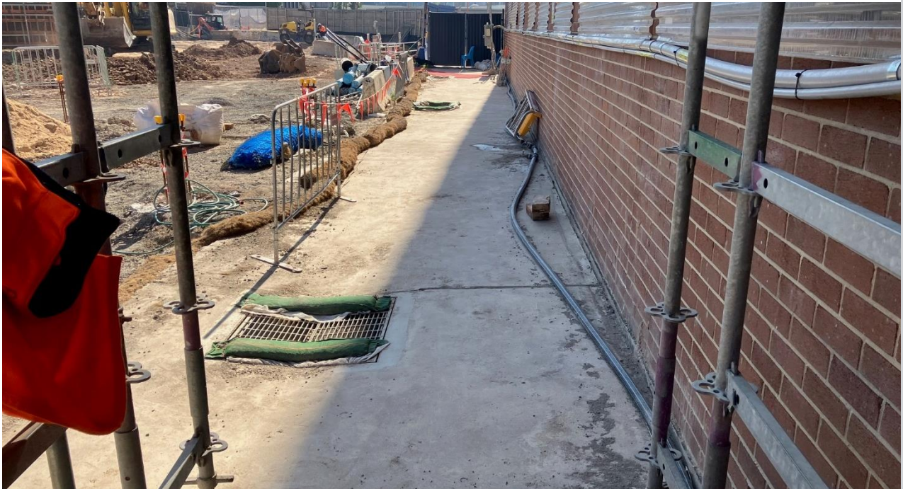
Protection of pit drains and controls; potable water available
