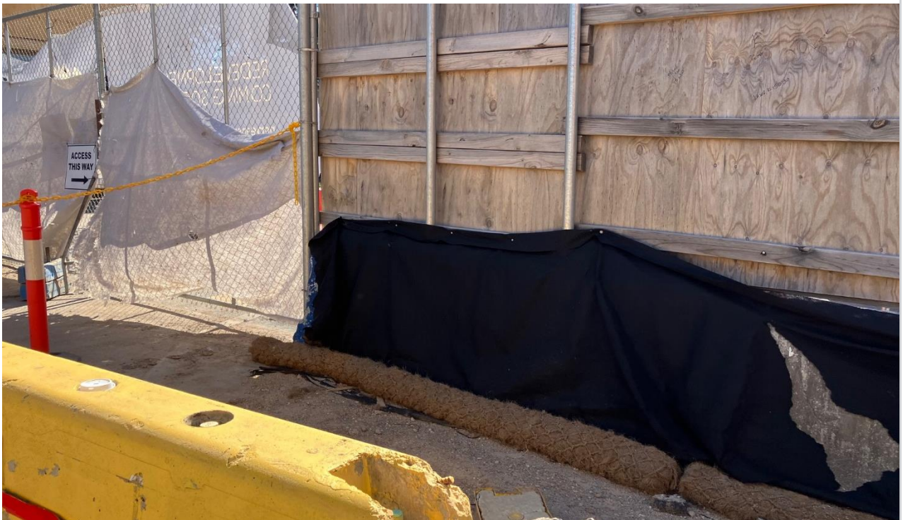
Hoarding and controls in place
