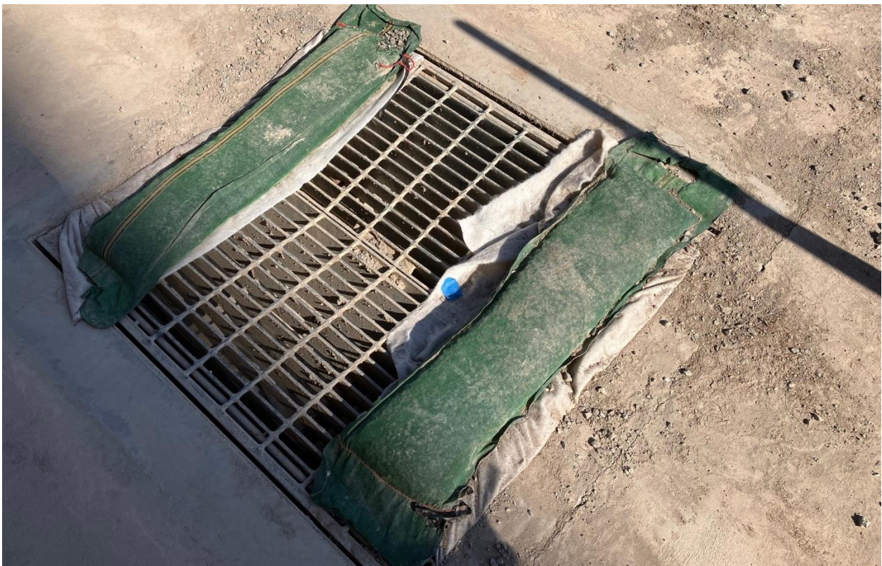
Protection of pit drains appeared well maintained
