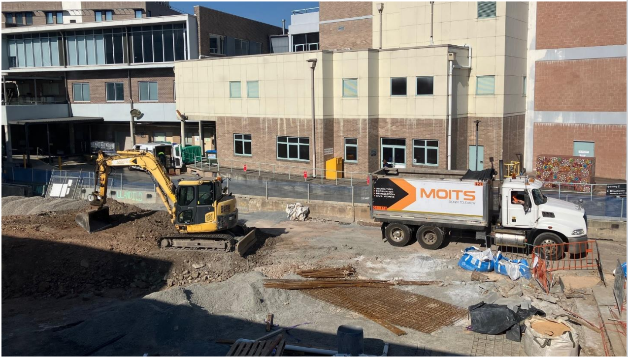
Loading dock works progressing
