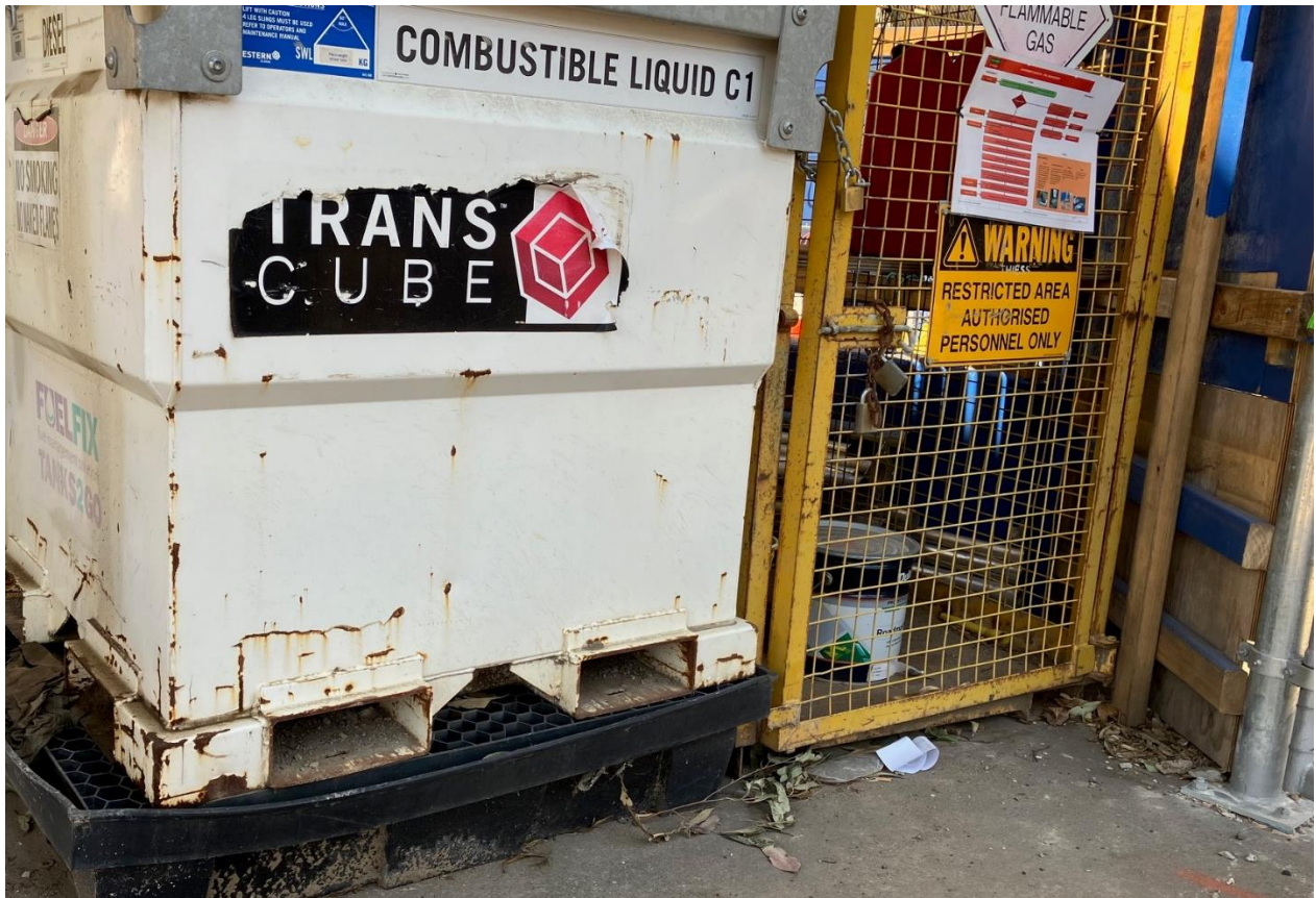
Bunded storage for hazardous materials.
