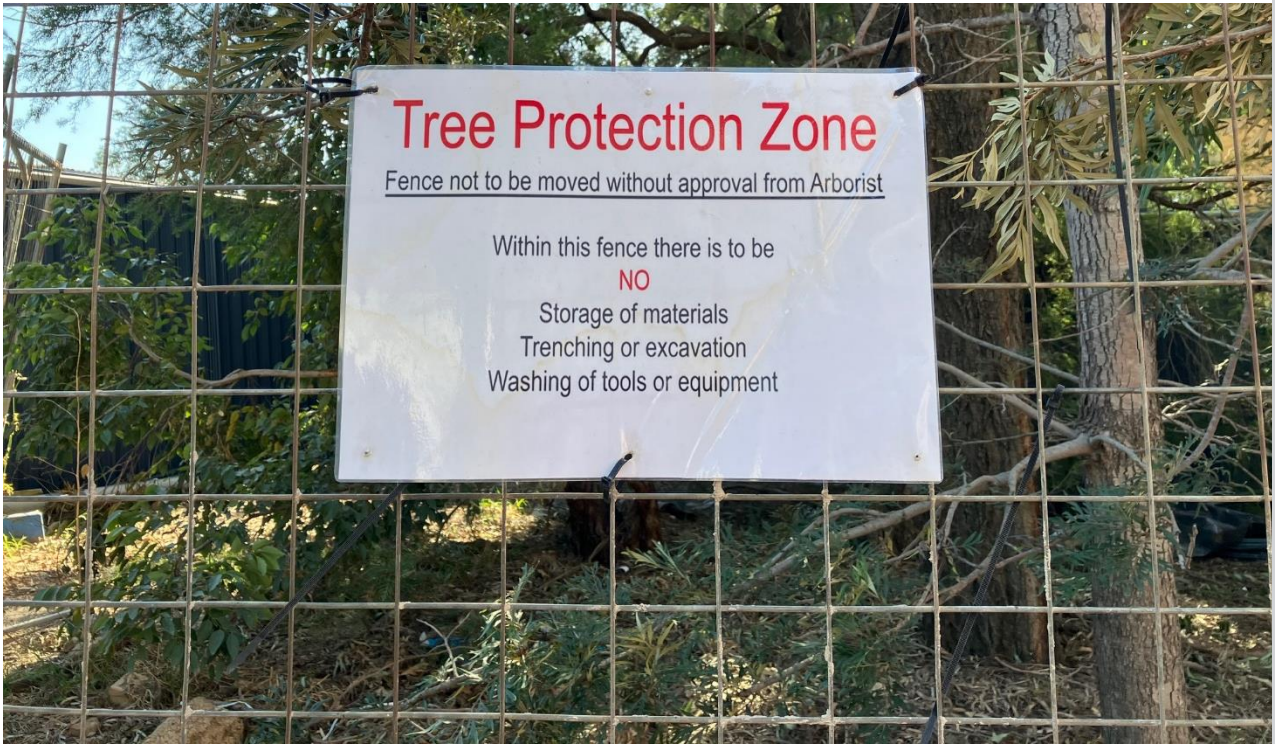
Tree Protection Zone (TPZ) signage
