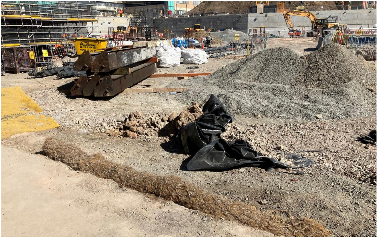
Areas stabilised throughout the site
