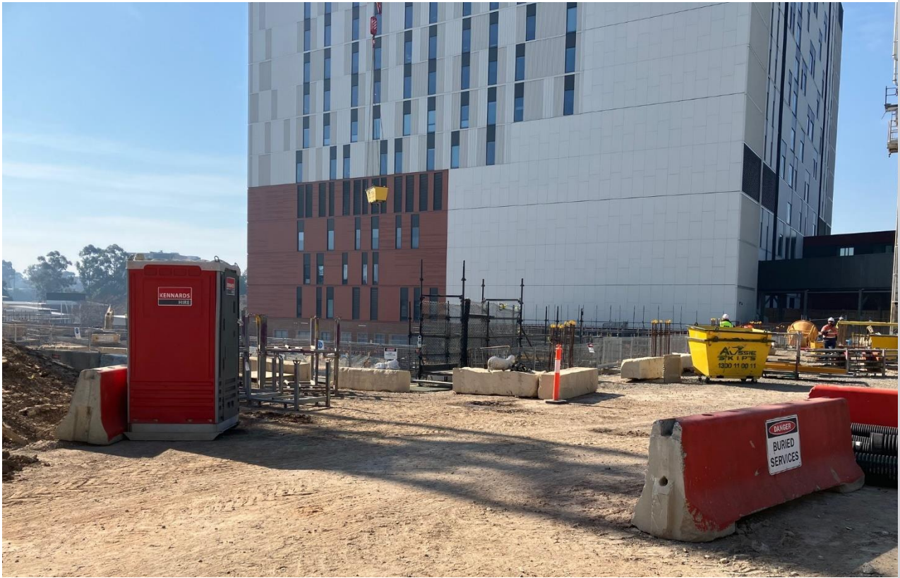
Generally good housekeeping observed on site
