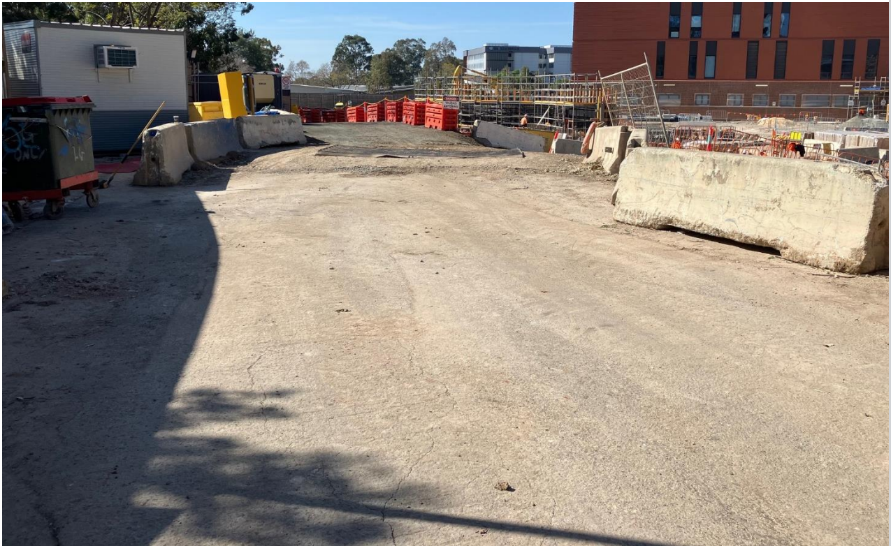
Heavy vehicle access. Area stabilised with rumble grid installed.
