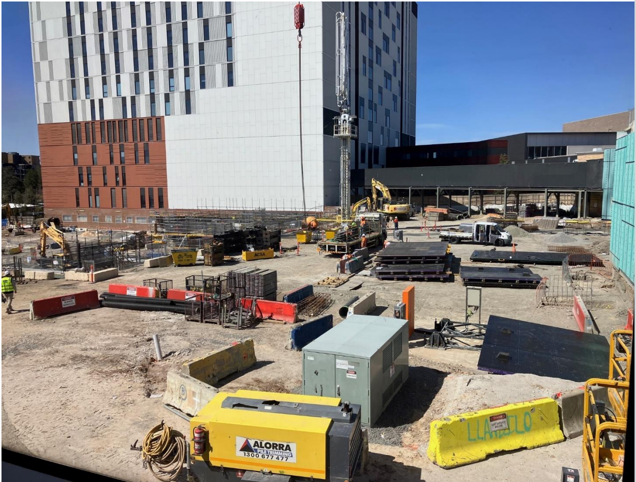
View point of site showing overall good housekeeping.
