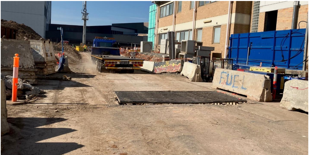
Rumble grid installed with areas stabilised.
