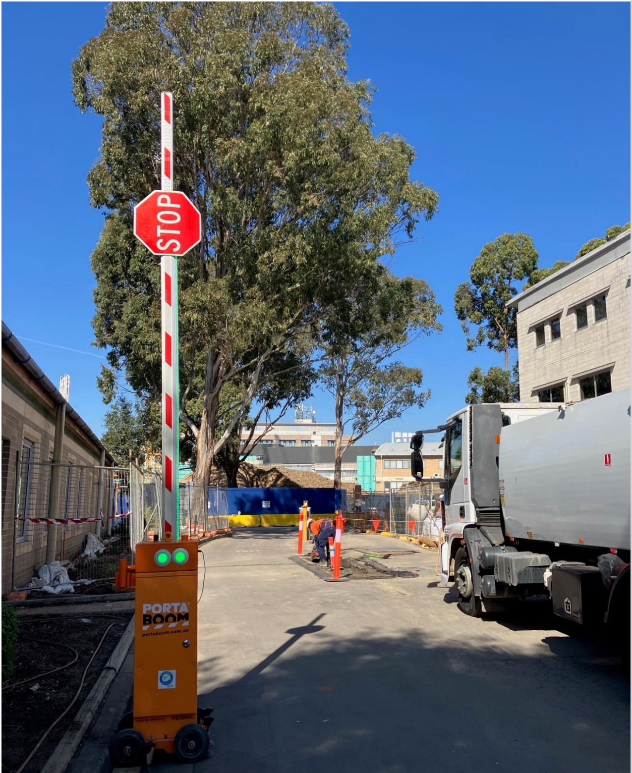
Traffic controls in place with boom gate operated by traffic controller.
