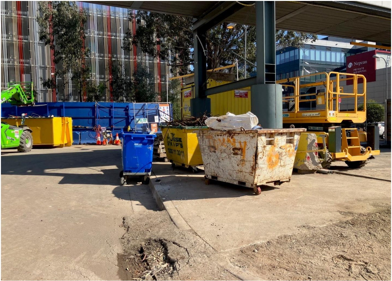
Some waste bins noted to be full however weekly bin collection occurring.
