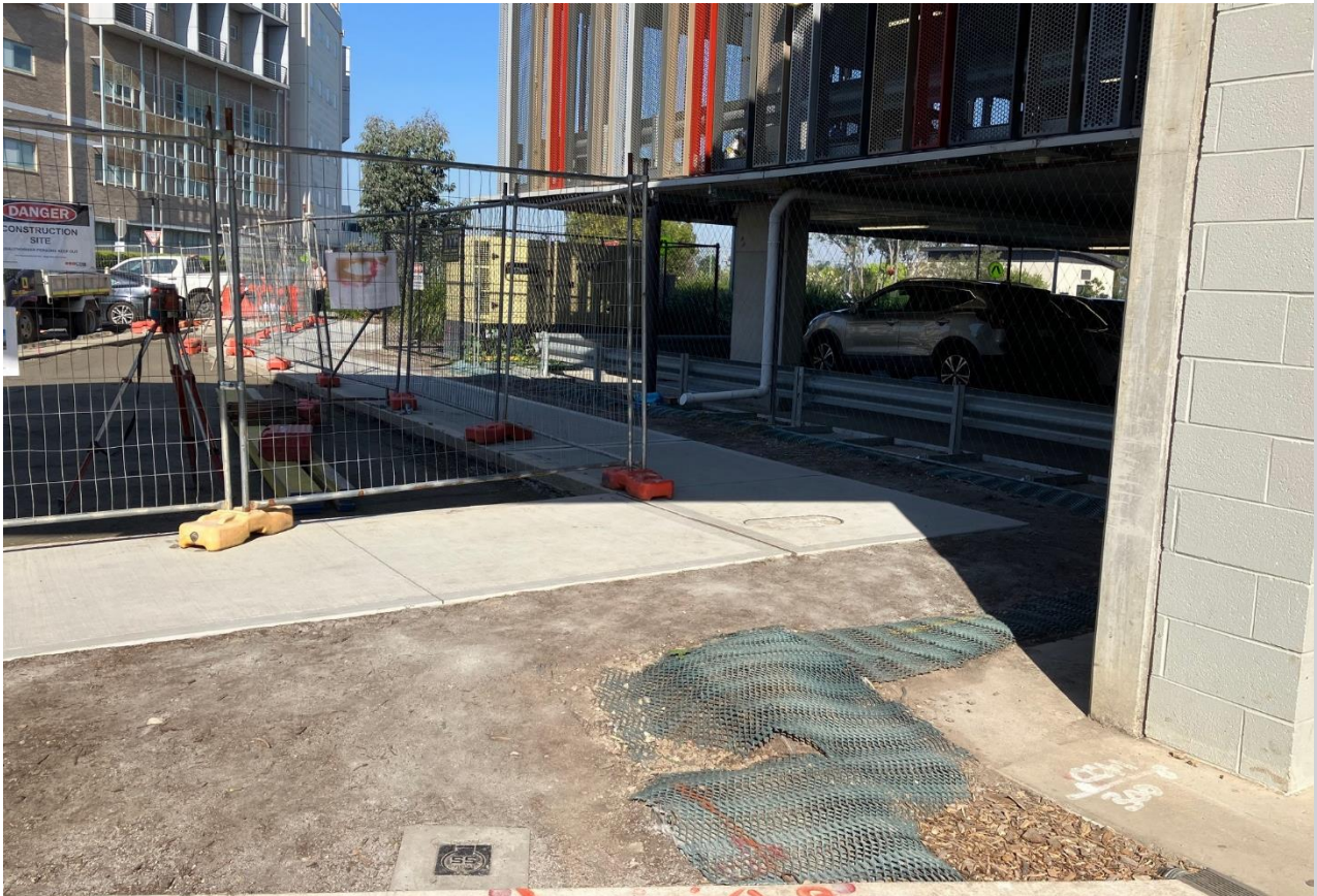
Pedestrian access kept clear adjacent to Car Park 1.
