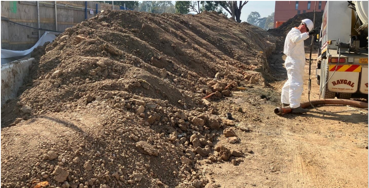
Vac truck being used during non-destructive borrow pit investigations
