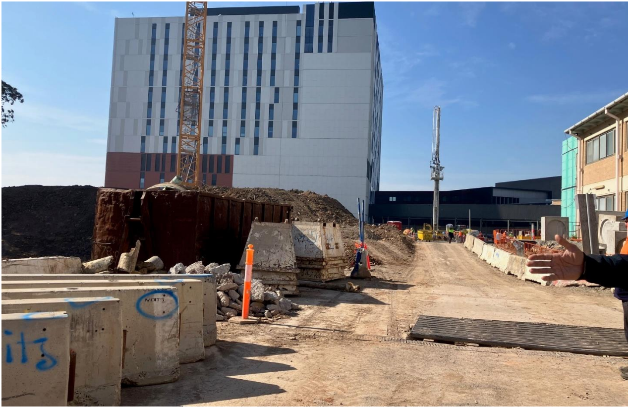
Materials observed to be neatly stored and separated by type.
