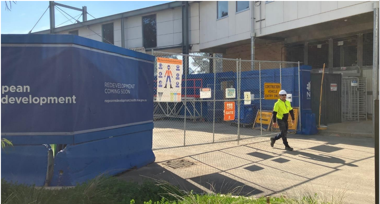
Secured access adjacent to link bridge.
