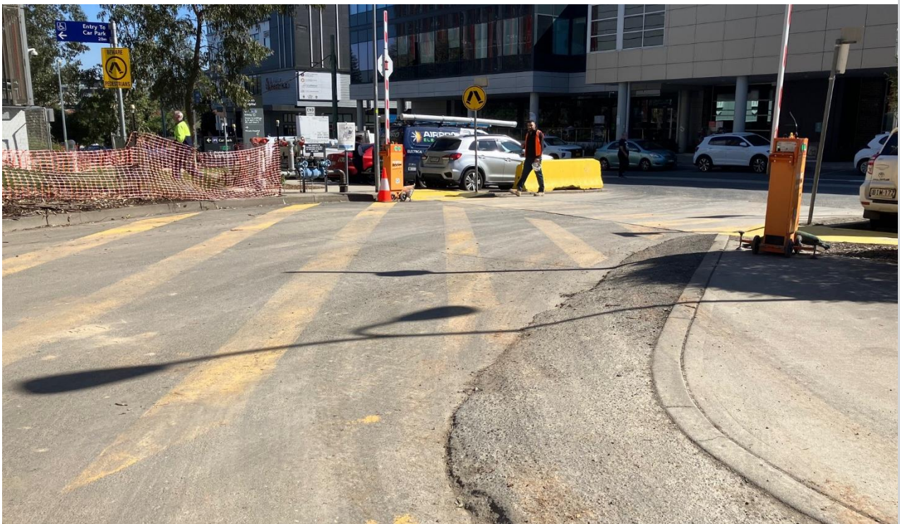
Traffic controls in place at Barber Avenue
