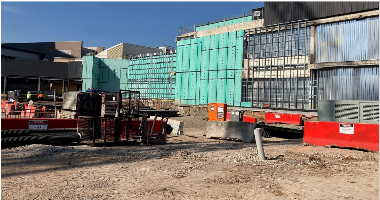
Façade underway at North Block (Stage 3 works)
