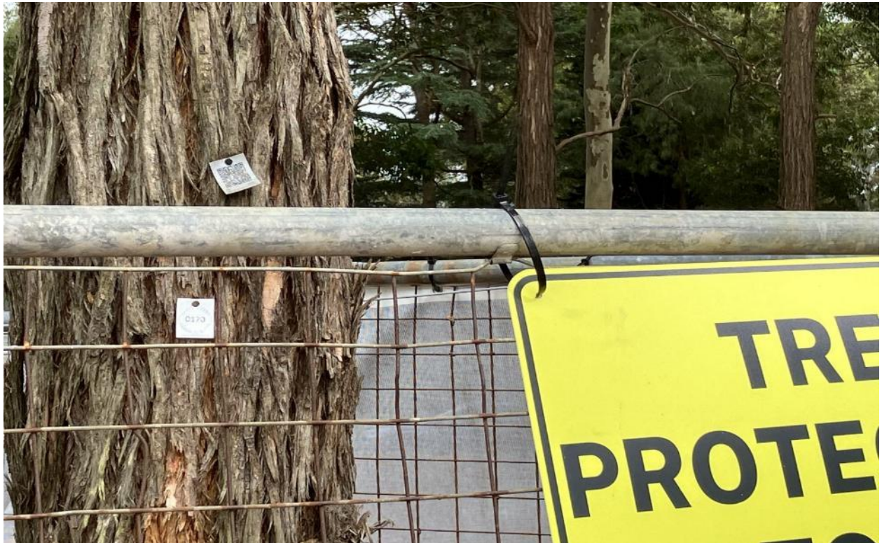
Retained trees marked with green ribbon and have unique number identifiers and QR code.
