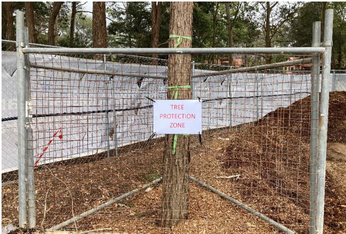
Closeout (OBS-02): Tree protection sign installed to close out OBS-02.
