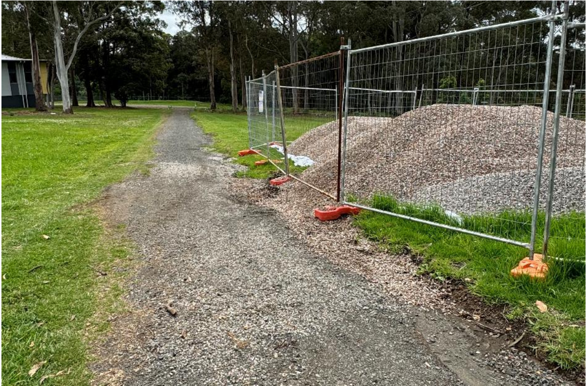
Closeout (OBS-05): The pathway has been cleared to close out OBS-05.
