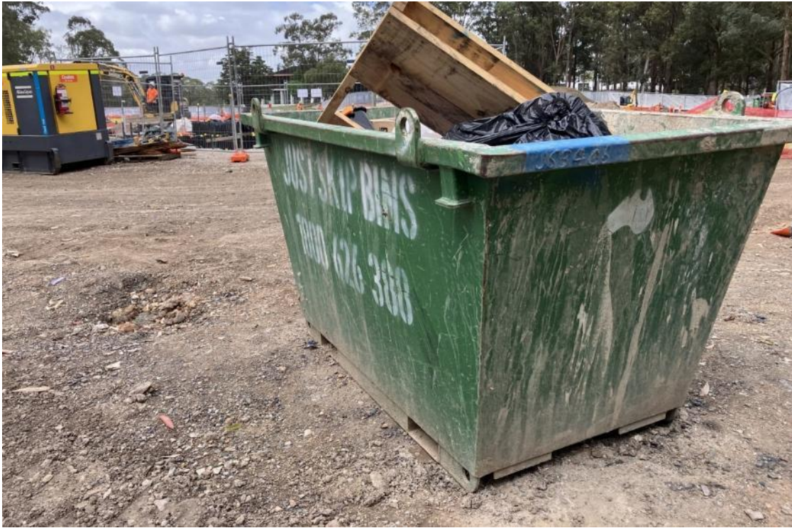
Skip bins available throughout the site.
