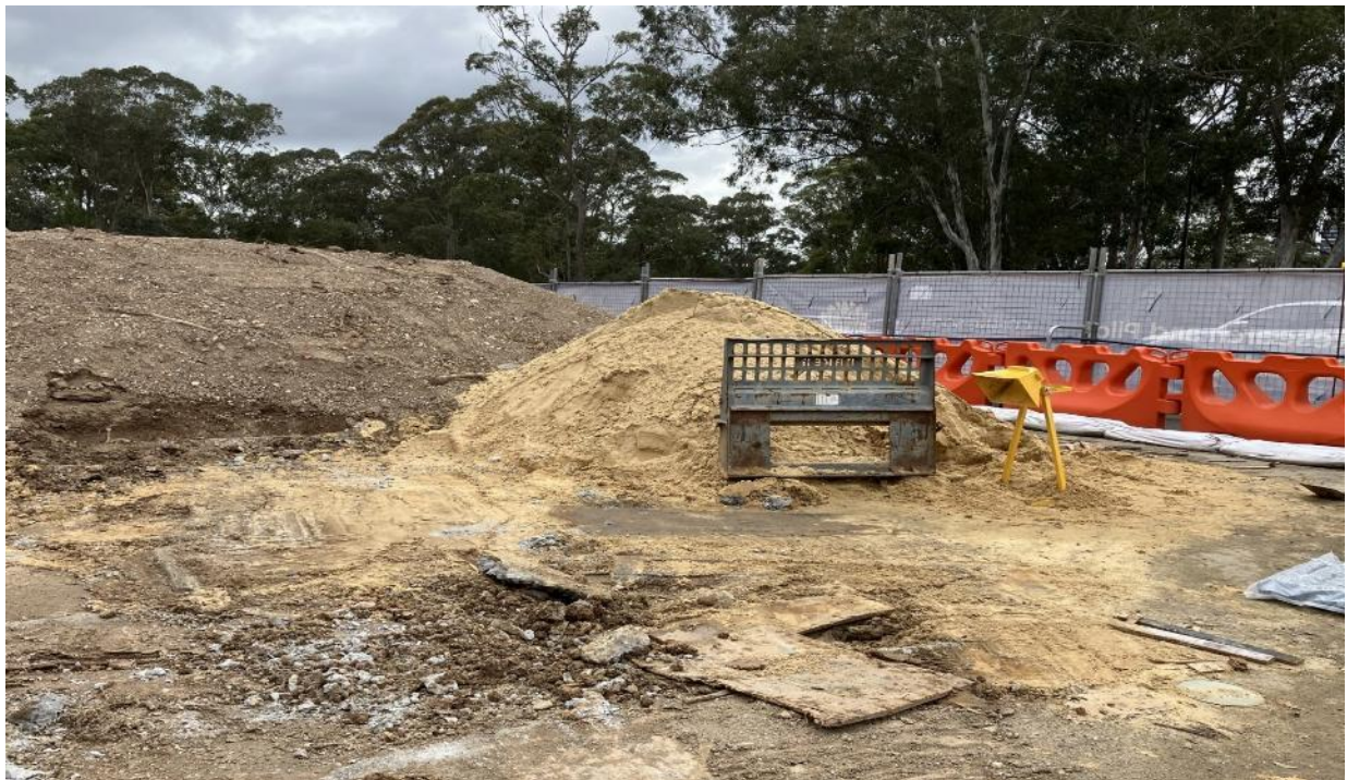
Materials stockpiled by type.
