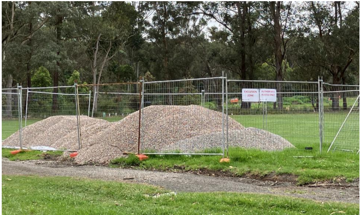
OBS-05: Stockpile area sitting outside site boundary was encroaching onto pathway.
