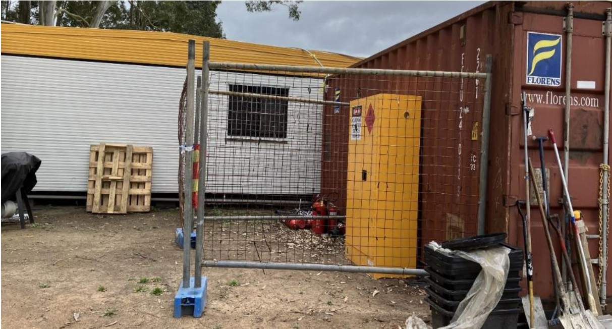
OBS-01: The spill kit was not located in close proximity to the hazardous chemicals shed and generator.
