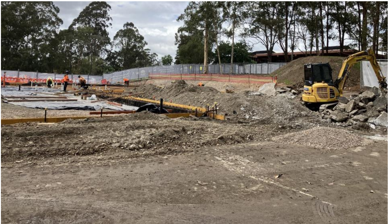
Construction activities in progress with no dust observed.
