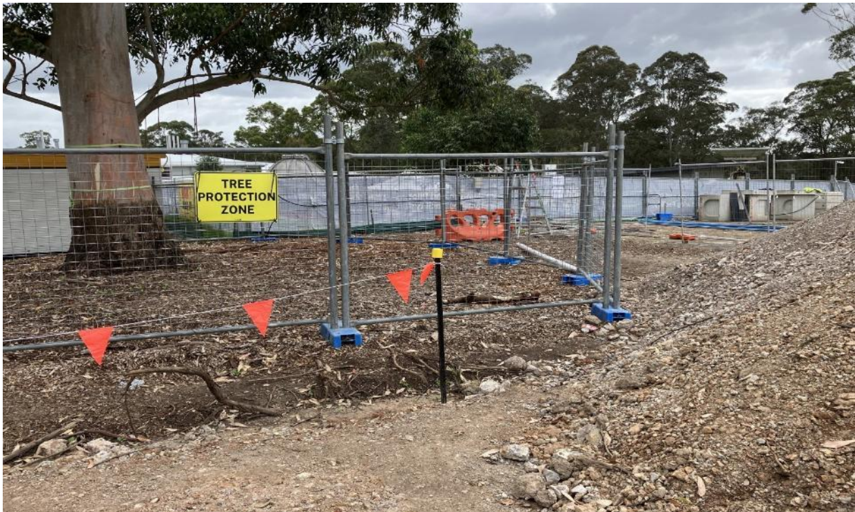
Fenced tree protection zones installed throughout the site.
