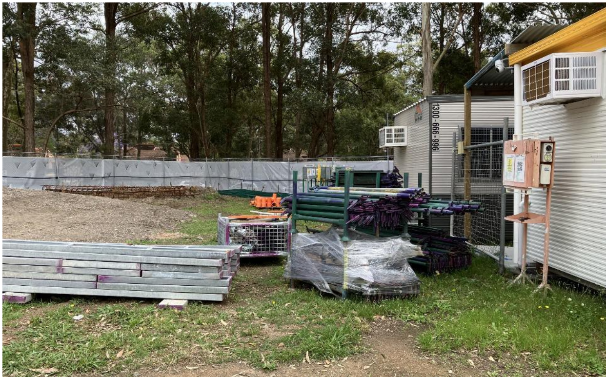
Site Laydown Area.
