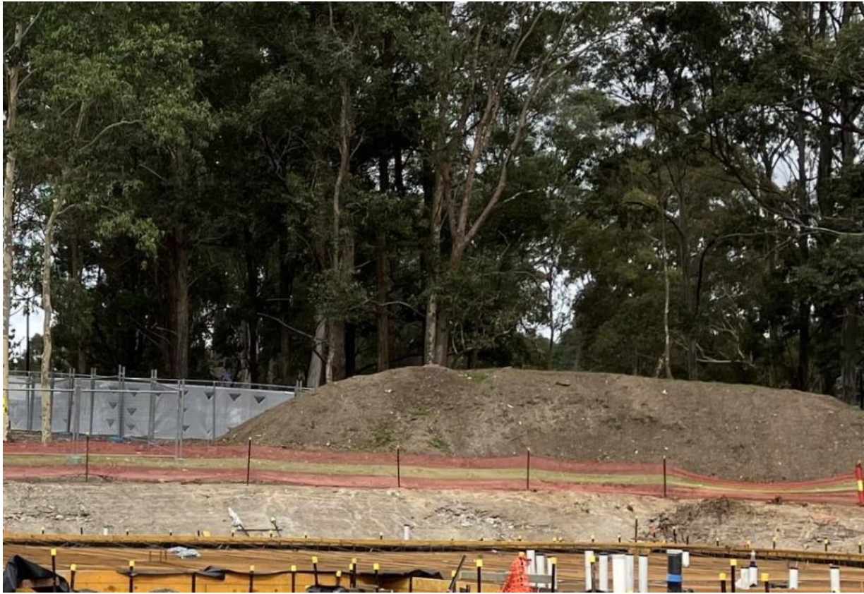
Topsoil stockpile clearly delineated.
