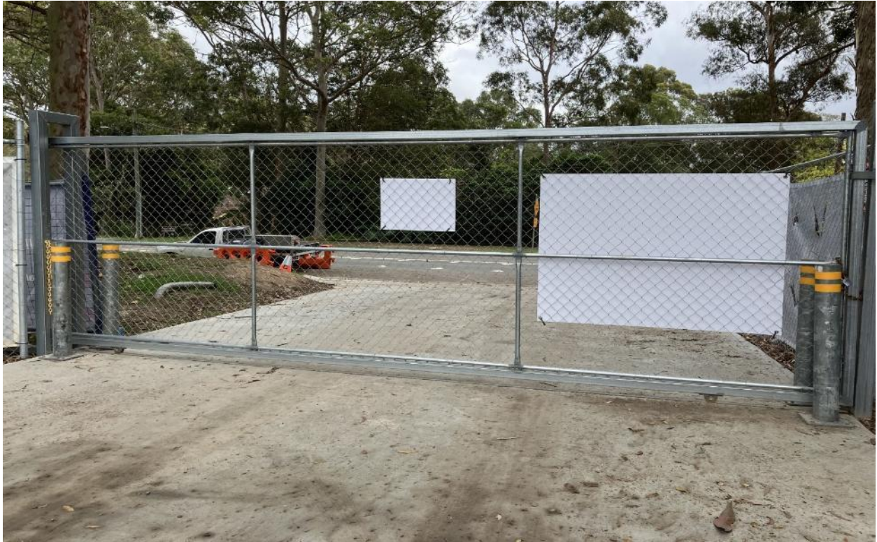
Site entrance locked and secured.
