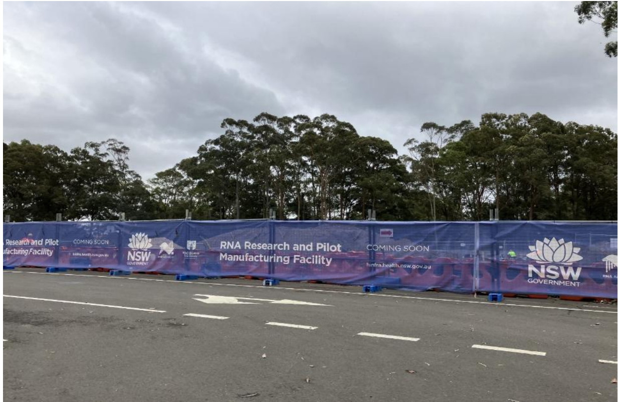
Shade cloth with ATF Fencing installed.
