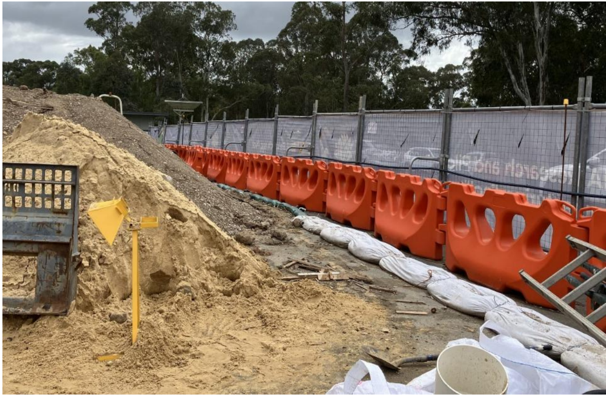
Sandbags in place at low point areas.
