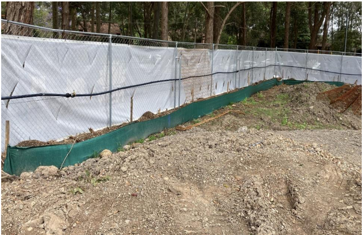
Sediment fence installed at low point areas.
