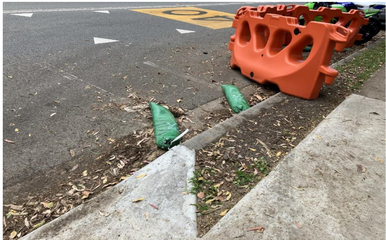
Closeout (OBS-03): Sandbag replaced to close out OBS-03.
