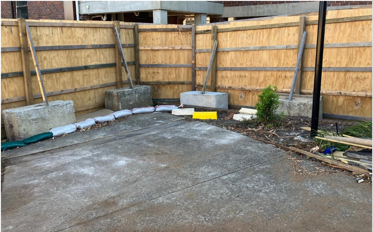
Hoarding and sandbags in place at Cleaners Building site.
