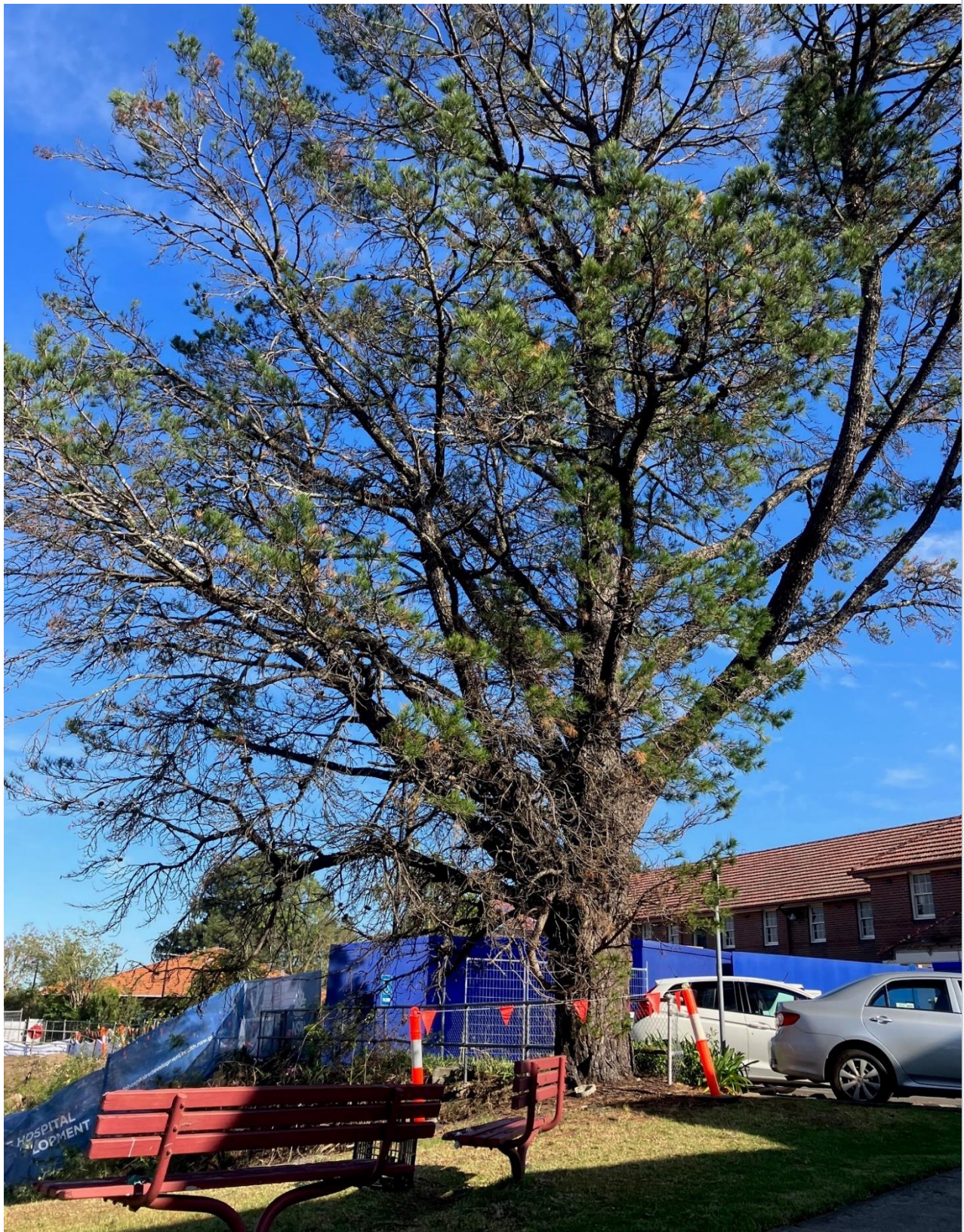
Tree retained under Milestone 3, however this will be removed at a later stage in the development.
