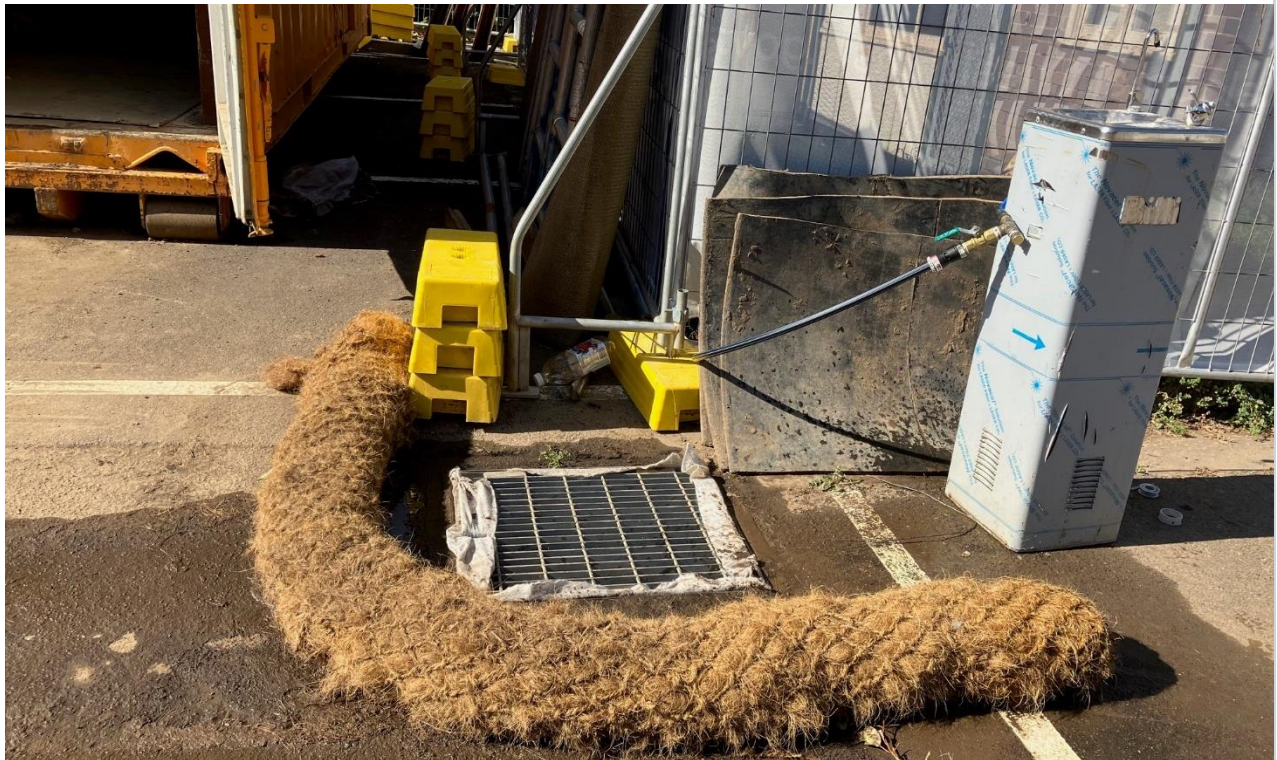
Protection of pit drain at Chatterly site
