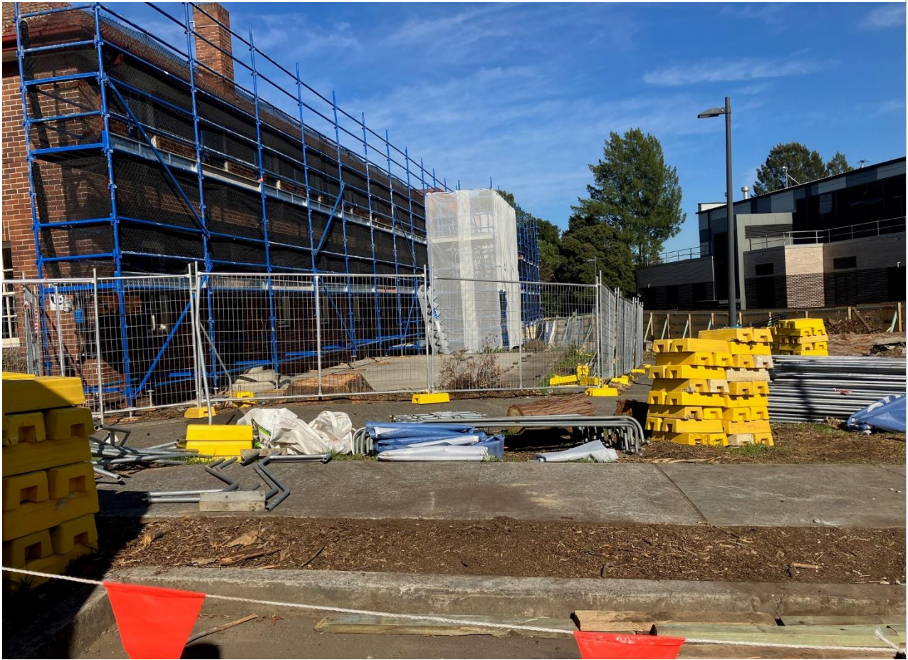
Preparations for demolition of the Chattery
