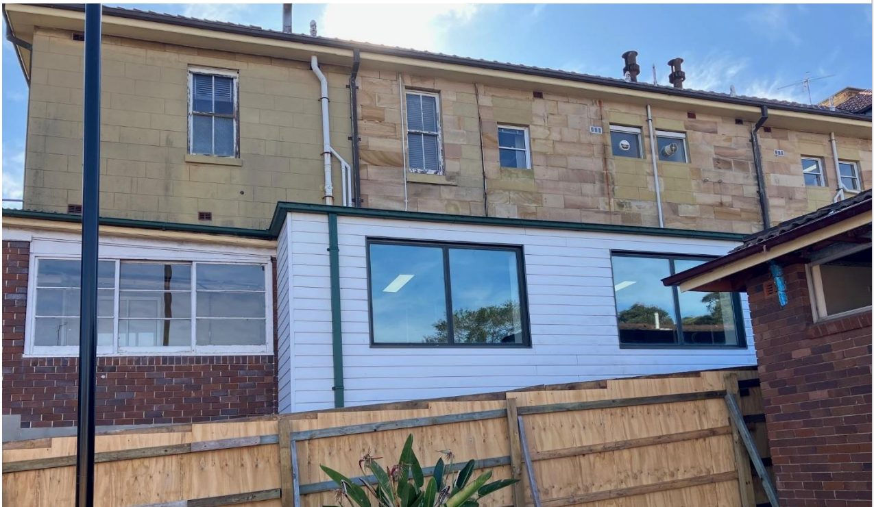
Denistone House and enclosed pedestrian walkway, Cleaners Building site.
