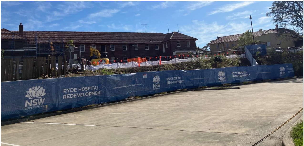
Carpark at Southern boundary adjacent to Chatterly site clean and clear of obstacles.
