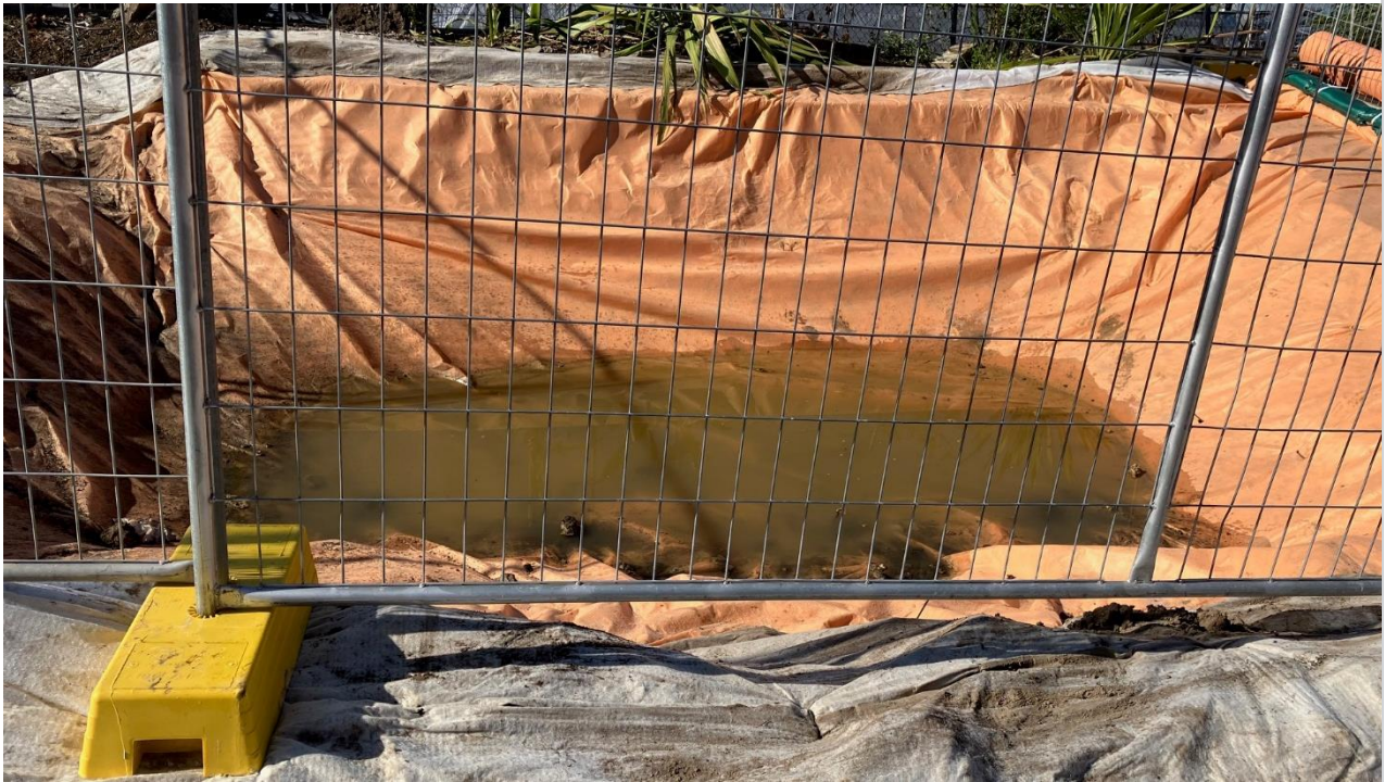
Sediment basin installed at Chatterry site
