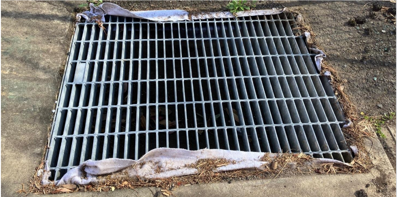
Protection of pit drains throughout the site
