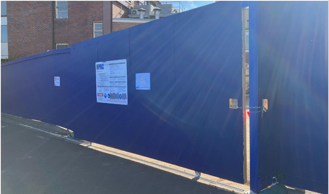
Secured hoarding with signage within hospital grounds.
