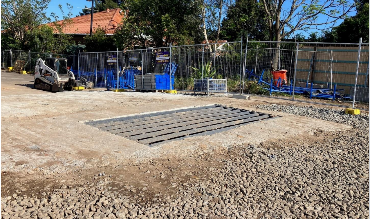
Rumble grid installed. Hardstand and rocks in place for stabilisation.
