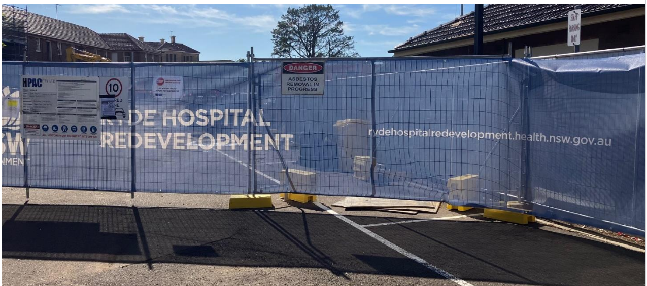
ATF with shade cloth and project signage
