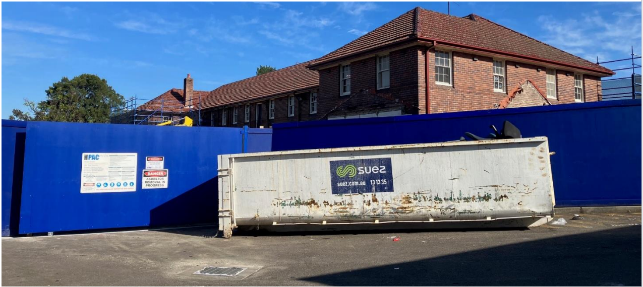
Hoarding installed within hospital grounds at Chatterly Building.
