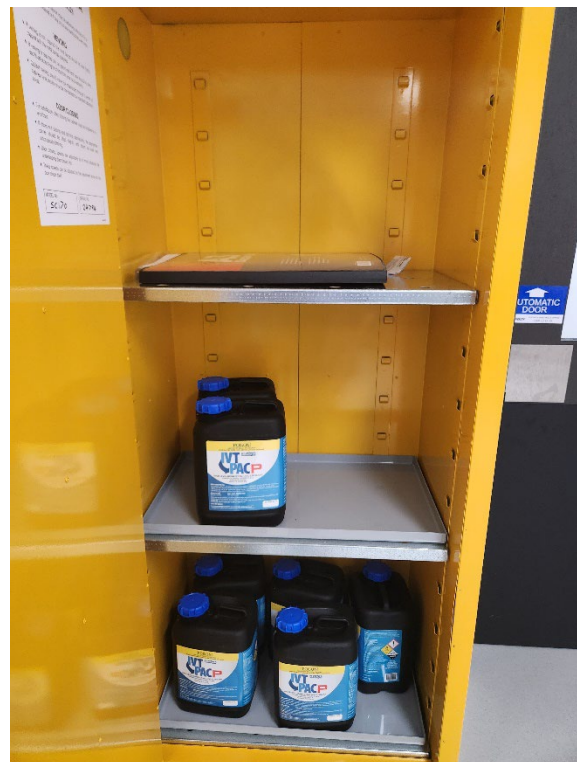
CSSD flammable liquids (provided by TSH).
