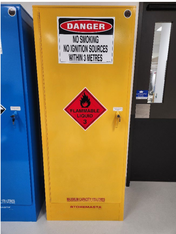
CSSD flammable liquid cabinet (provided by TSH).
